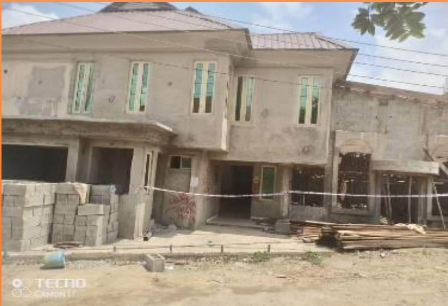
5. On going construction at No 122, Lateef Adekola Close, Oshodi
