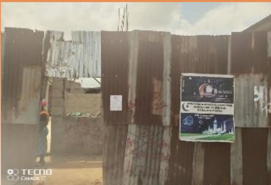
6. On-going development No 44, Eyinogun Street, Oshodi
