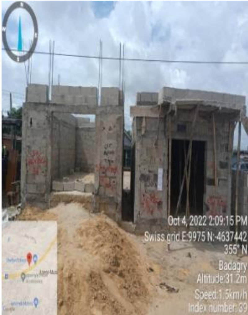
COMMERCIAL DEVELOPMENT ALONG LAGOS EXPRESSWAY, ILE EPO BUSTOP, ARAROMI OLORUNDA LCDA.
