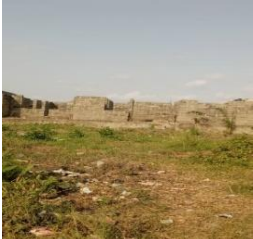
OFF LAGOS BADAGRY EXPRESSWAY , AGOGO-IGBALA OLORUNDA LCDA
