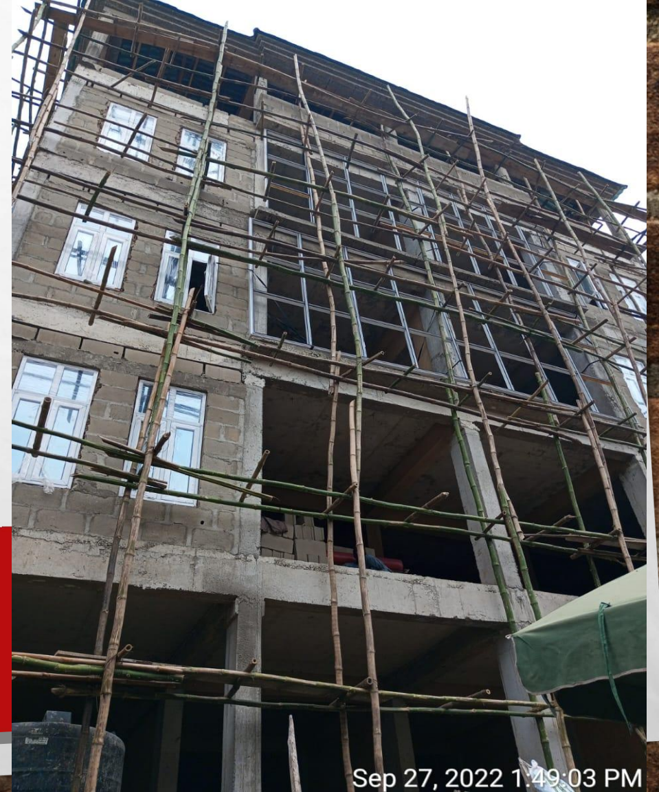
Location: 56, IDUMAGBO AVENUE, IDUMOTA, LAGOS ISLAND. Stage: FINISHES
