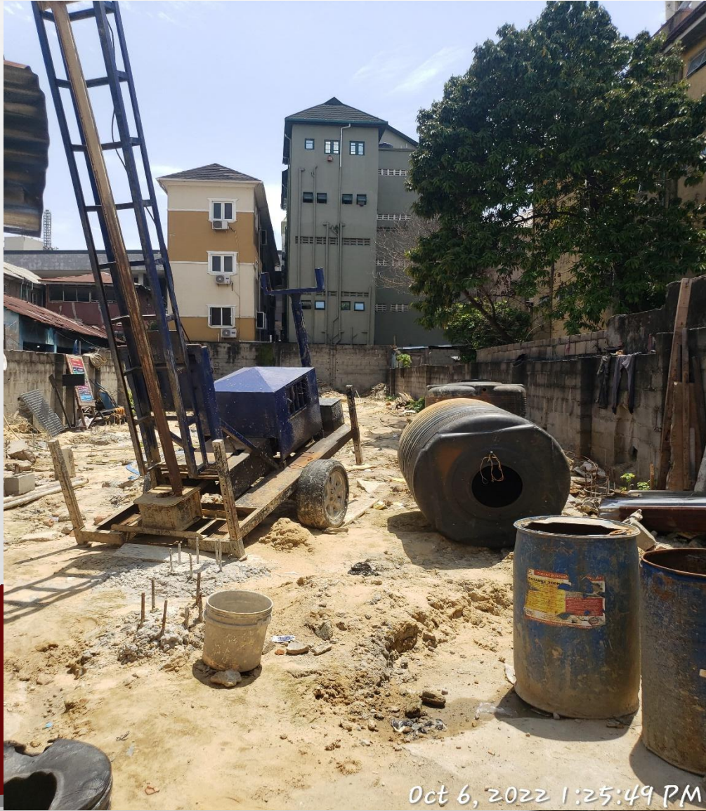
Location: 170, Bamgbose Street, Lagos Island, Lagos.
