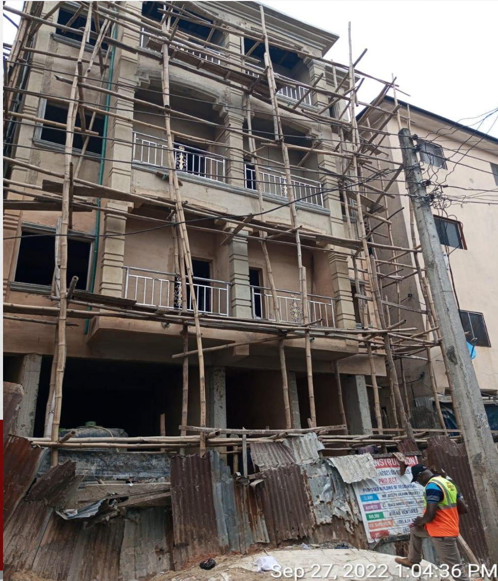
Location: 25, ISALE AGBEDESTREET Stage: FINISHES
