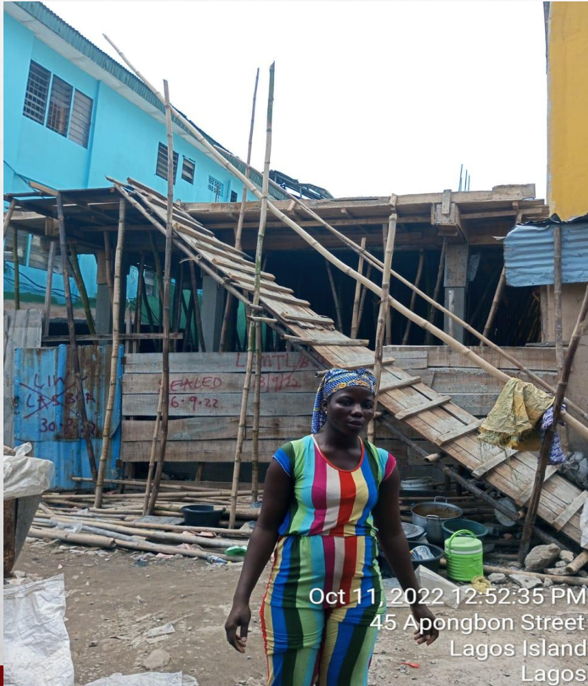
Location: 77 APONGBON STREET, LAGOS ISLAND. Stage: FIRST FLOOR SLAB FORMWORK/REINFORCEMENT
