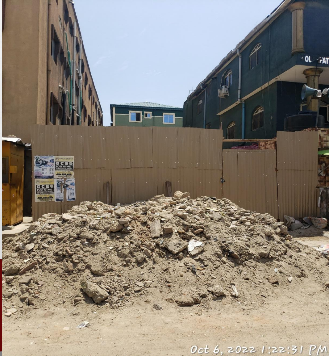
Location: 182, Bamgbose Street, Lagos Island, Lagos
