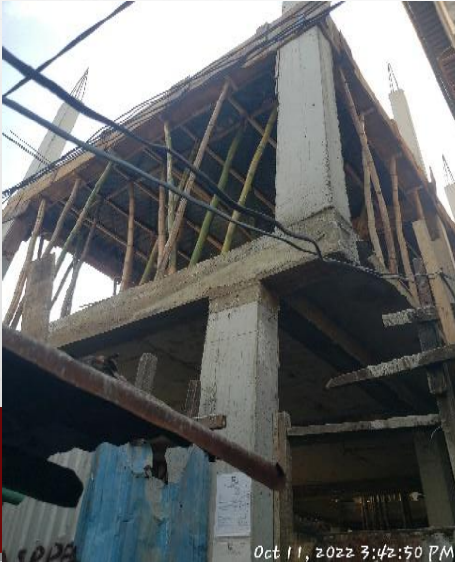
Location: 66, Lewis Street, Lafiaji, Lagos. STAGE: SECOND SUSPENDED FLOOR SLAB
