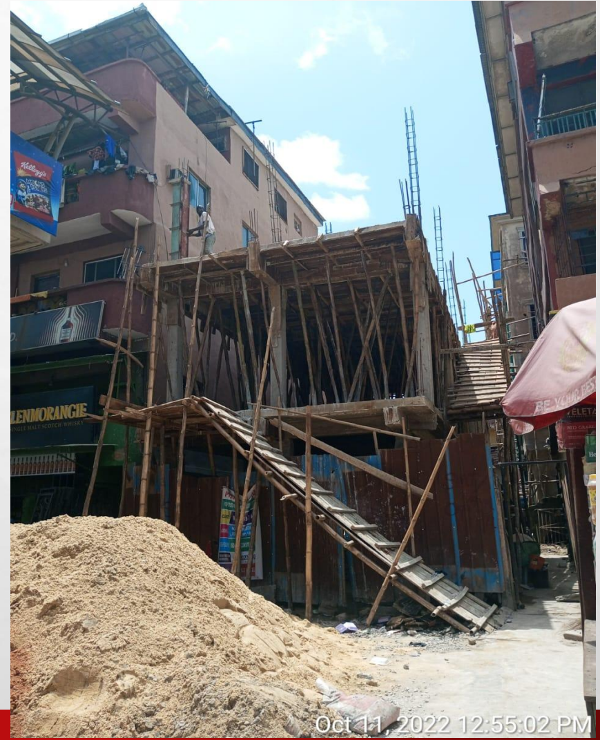
Location: 51 APONGBON STREET, LAGOS ISLAND. Stage: SECOND FLOOR COLUMN
