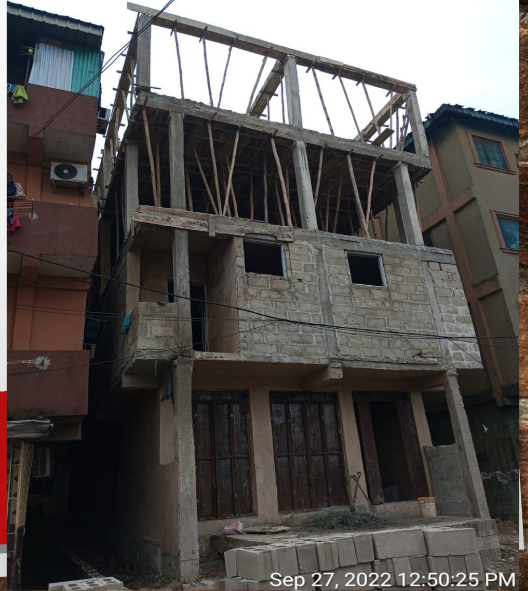
Location: 6, COLLINS STREET OFF BINUYO STREET Stage: ROOF BEAM
