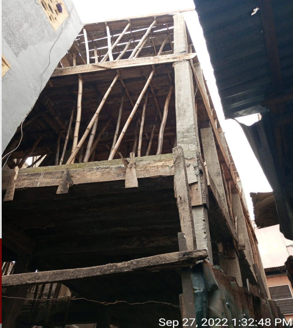
Location: 4, IBOMO STREET LAGOS ISLAND. Stage: THIRD SUSPENDED FLOOR SLAB FORMWORK
