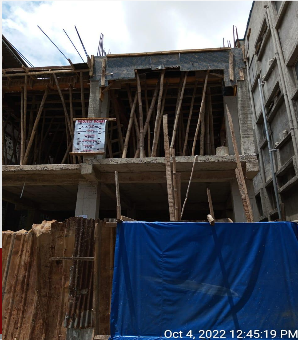
Location: 20 DOHERTY STREET LAGOS ISLAND Stage: SECOND SUSPENDED FLOOR FORMWORK
