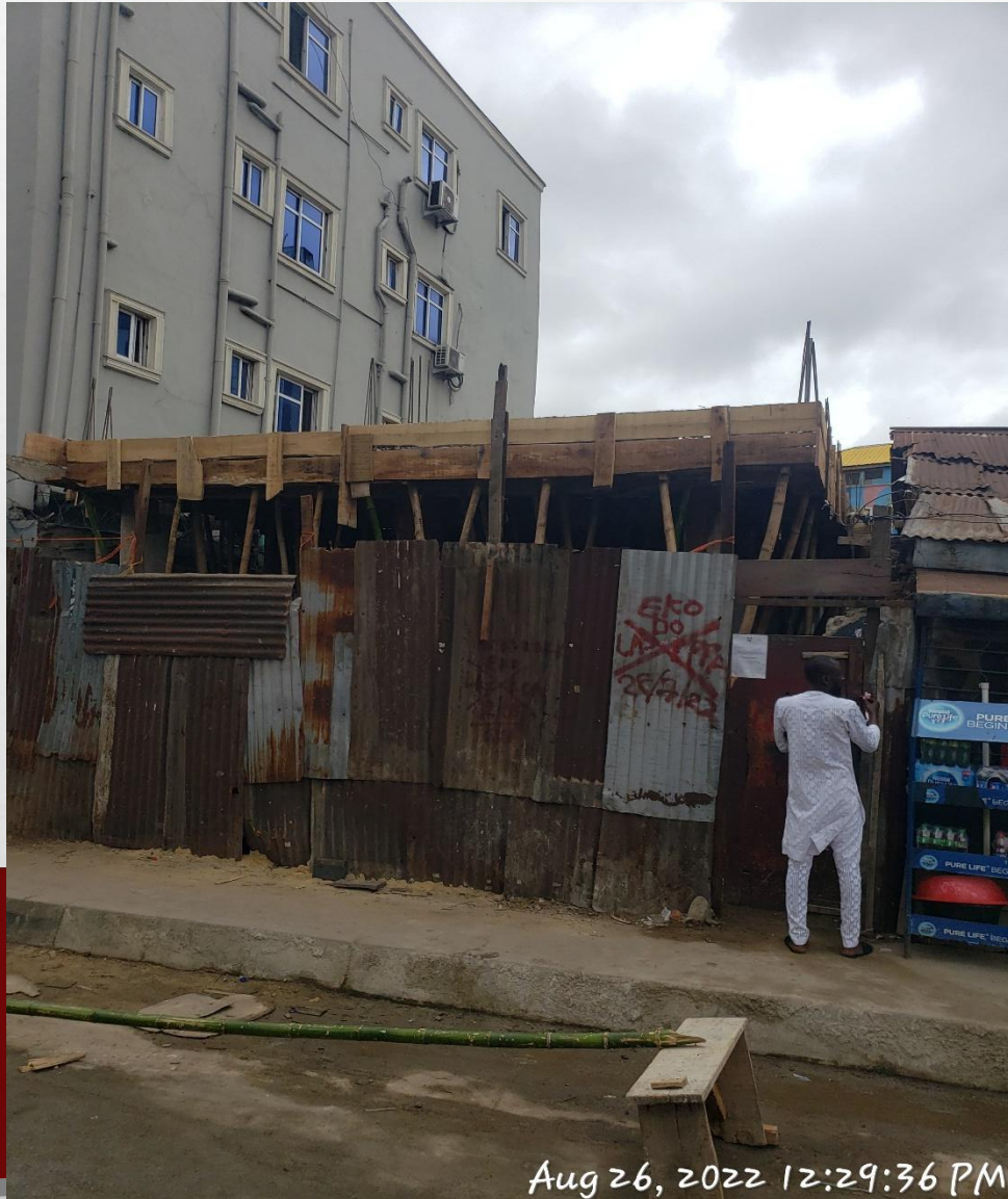
Location: 3, Campbell Street, Lagos Island, Lagos. STAGE: FIRST SUSPENDED FLOOR SLAB
