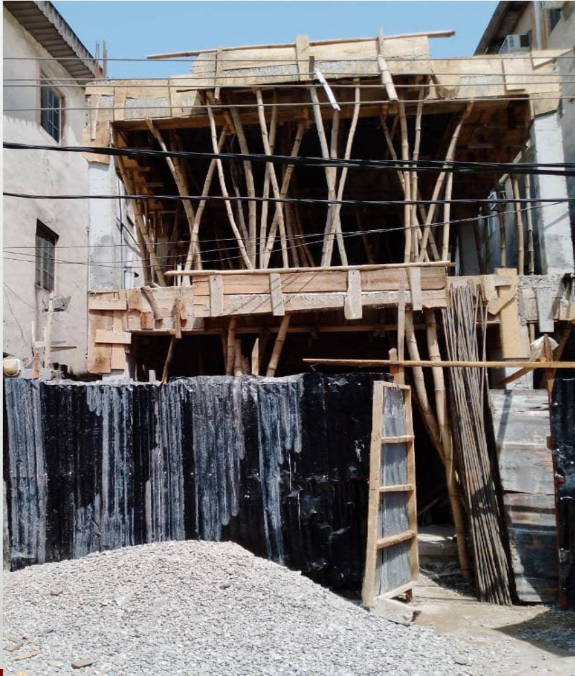
LOCATION: 141, IGBOSERE STREET, LAGOS ISLAND, LAGOS. STAGE: SECOND SUSPENDED FLOOR FORMWORK
