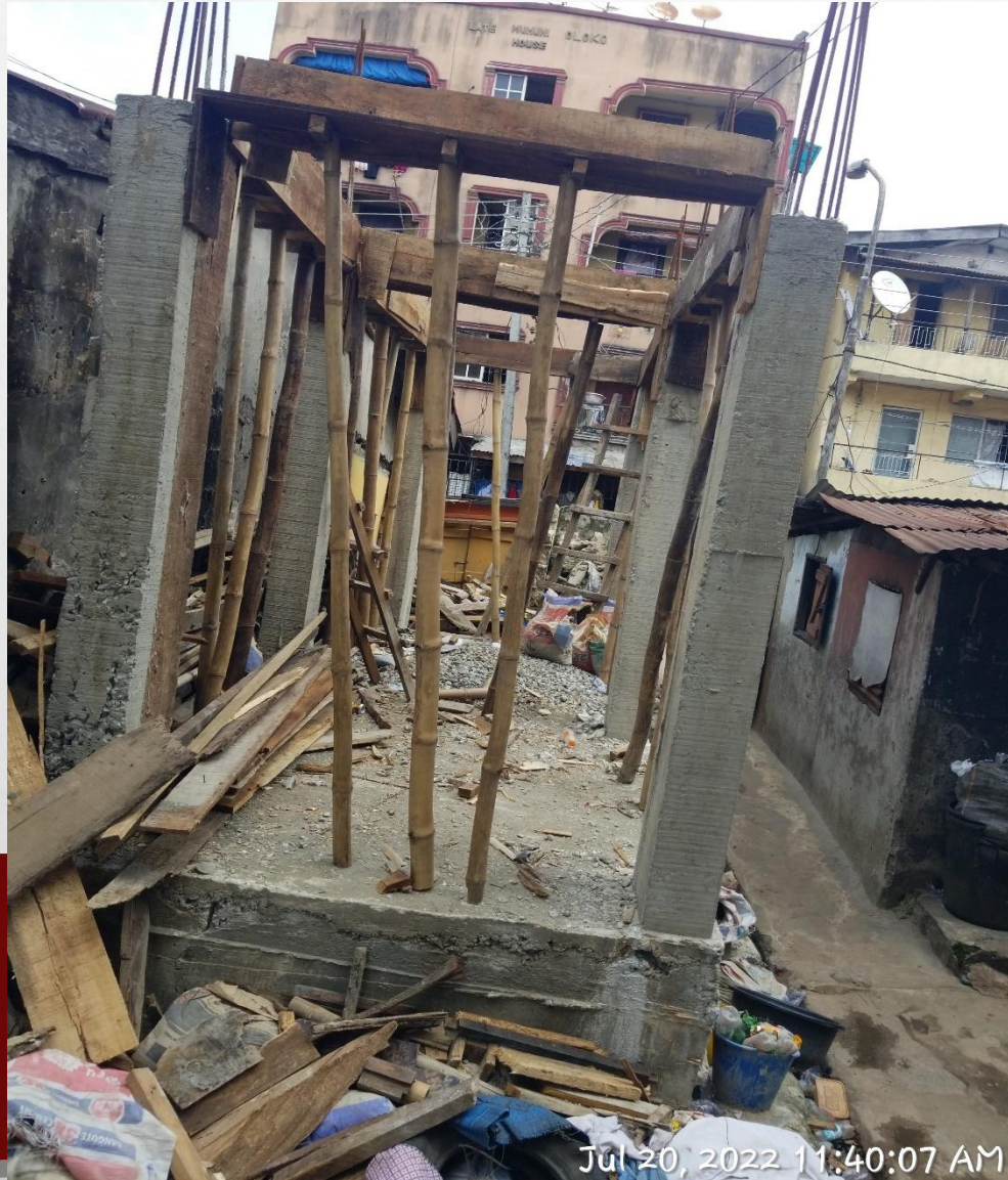
Location: 76, Glover Street, Lagos Island, Lagos. STAGE: GROUND FLOOR COLUMN
