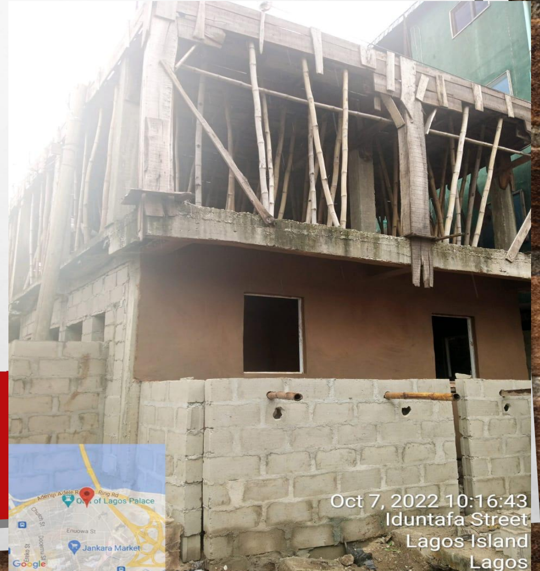
Location: 2, IDUNTALA STREET Stage: SECOND SUSPENDED FLOOR FORMWORK
