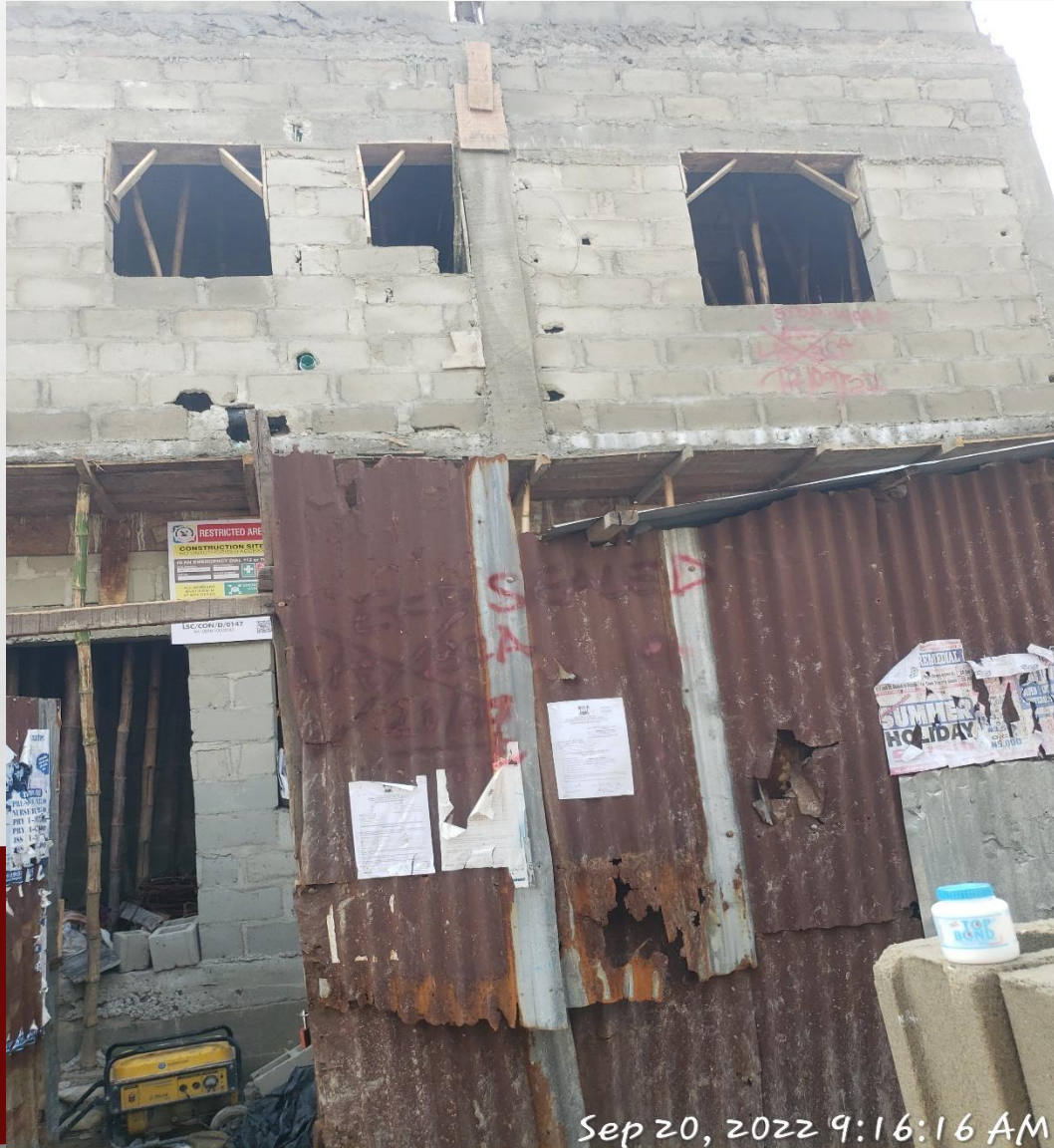
Location: 50, Alof Street, Lagos Island, Lagos. STAGE: SECOND SUSPENDED FLOOR REINFORCEMENT
