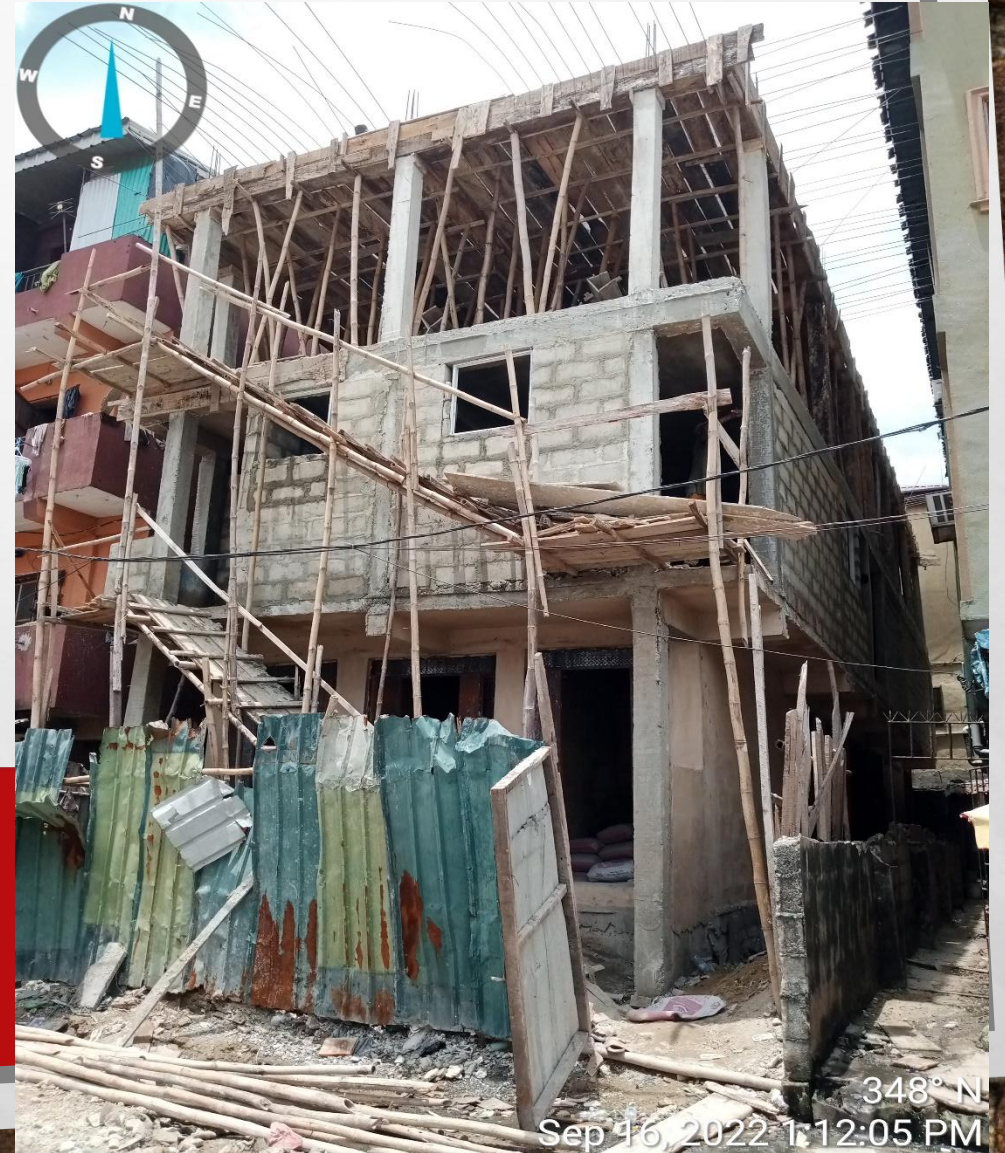
Location: 58, Tokunboh Street, Lagos Island, Lagos. STAGE: SECOND SUSPENDED FLOOR REINFORCEMENT
