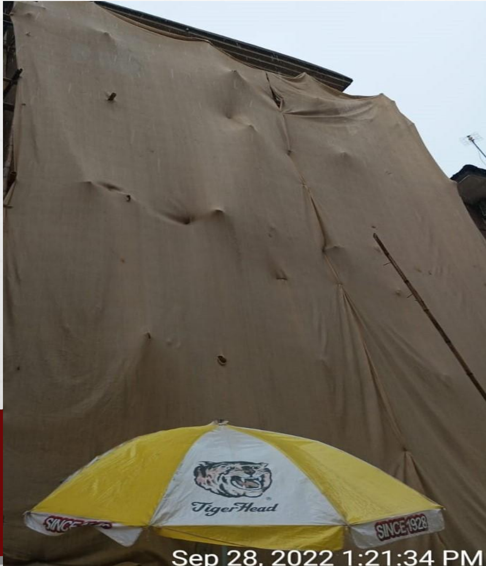
Location: 97B, DOCEMO STREET Stage: SECOND SUSPENDED FLOOR FORMWORK
