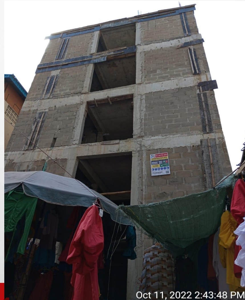
Location: 10 SANNI ADEWALE STREET , LAGOS ISLAND. Stage: PLASTERING
