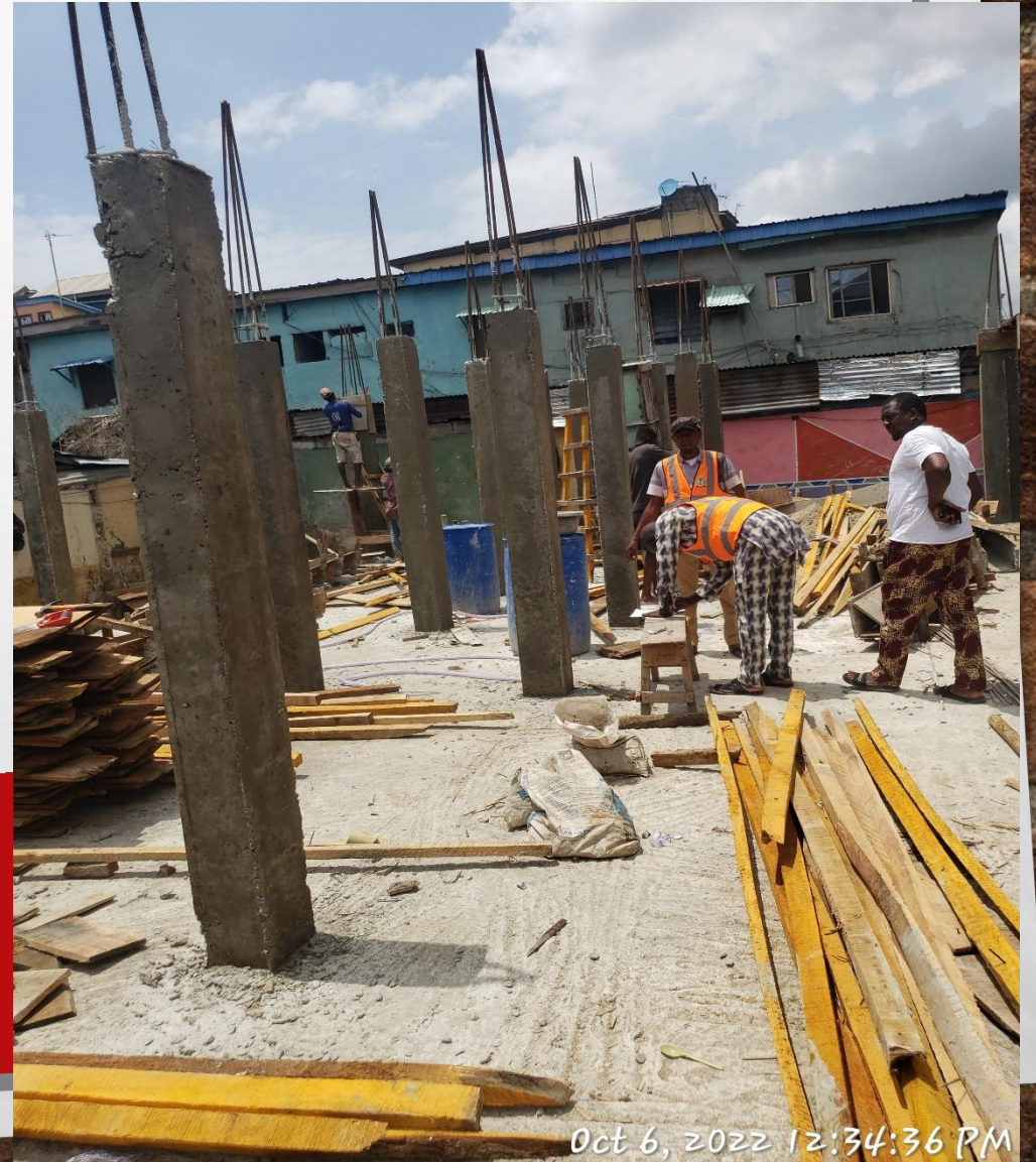
Location: 7, Dumare Street, Lagos Island, Lagos. STAGE: GROUND FLOOR COLUMN
