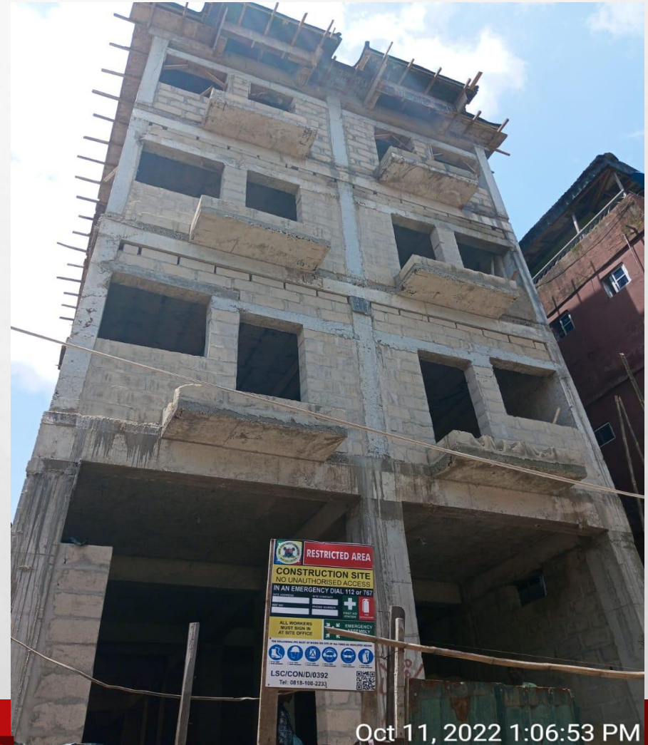
Location: 7 GRIFFIN STREET OFF ELEGBATA, LAGOS ISLAND. Stage: ROOFED
