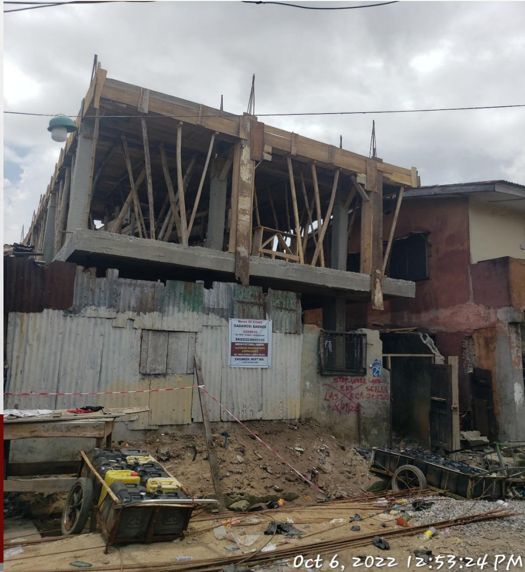
Location: 29, Patey Street, Lagos Island, Lagos. STAGE: SECOND SUSPENDED FLOOR FORMWORK
