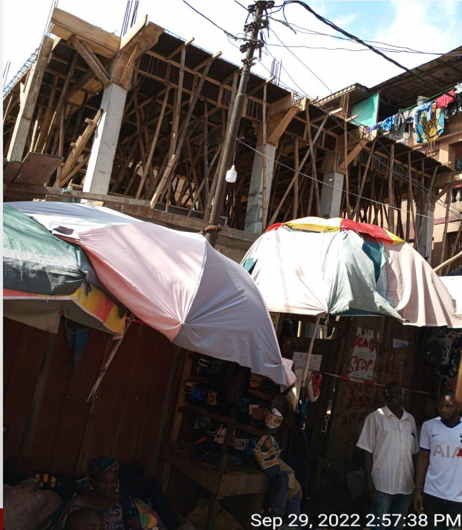
Location: 56 AGORO STREET LAGOS ISLAND. Stage: THIRD FLOOR SLAB FORMWORK
