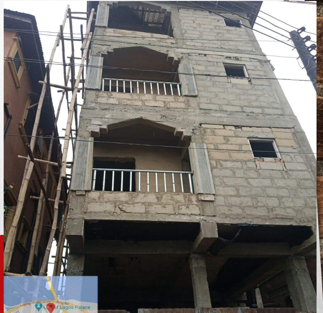
Location: 21 ONILEGBALE STREET LAGOS ISLAND Stage: FINISHES
