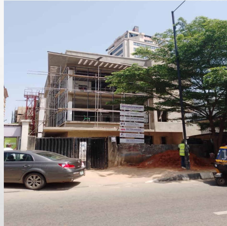
Location: 30, BROAD Street, Lagos Island, Lagos. STAGE: Roofing Ongoing
