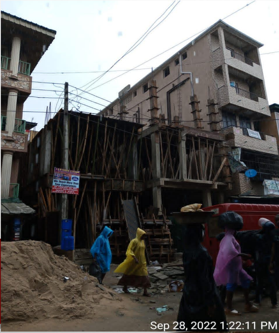
Location: 101 DOCEMO STREET Stage: SECOND SUSPENDE FLOOR COLUMN
