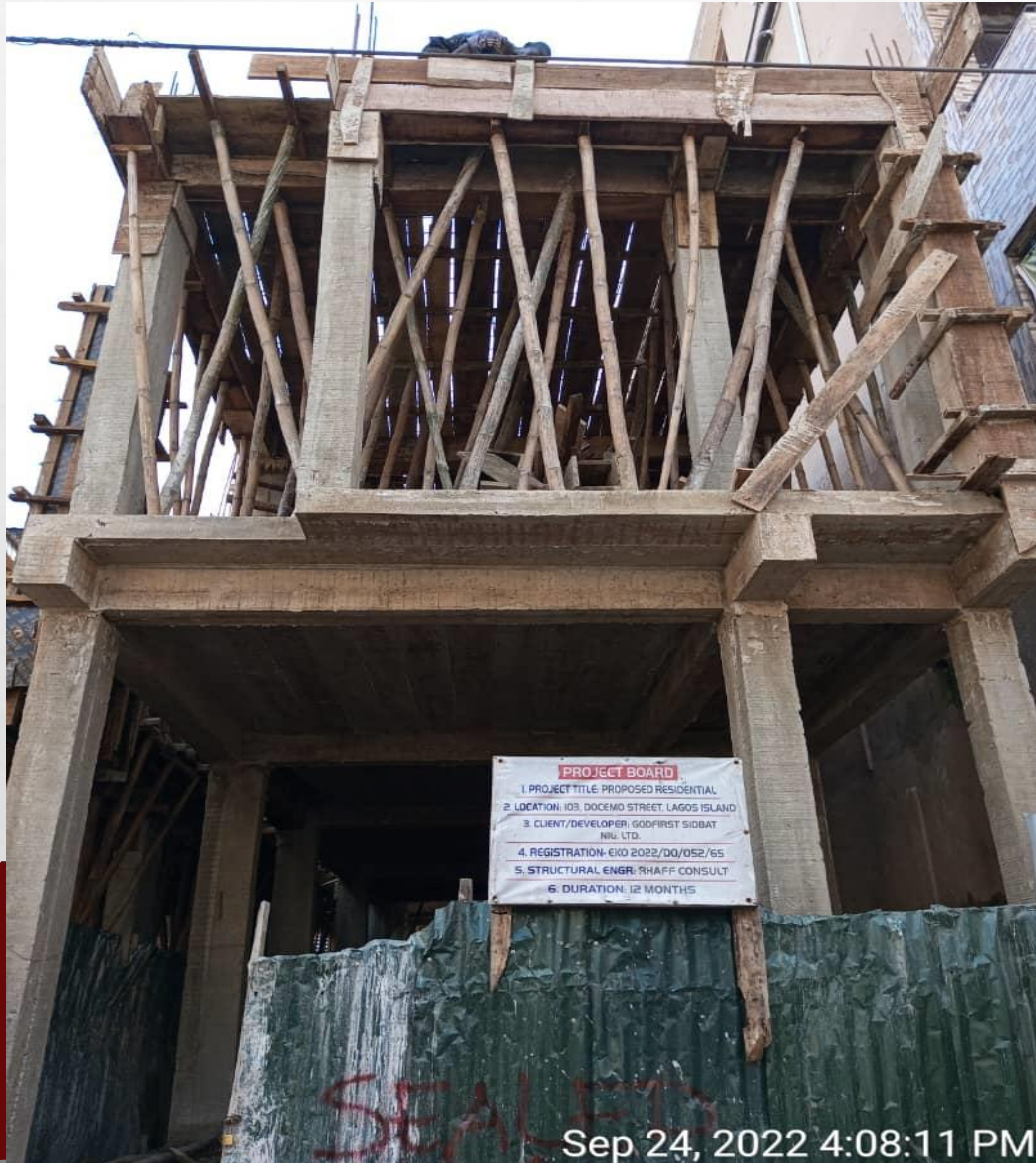
Location: 112 DOCEMO STREET LAGOS ISLAND Stage: THIRD FLOOR SLAB FORMWORK
