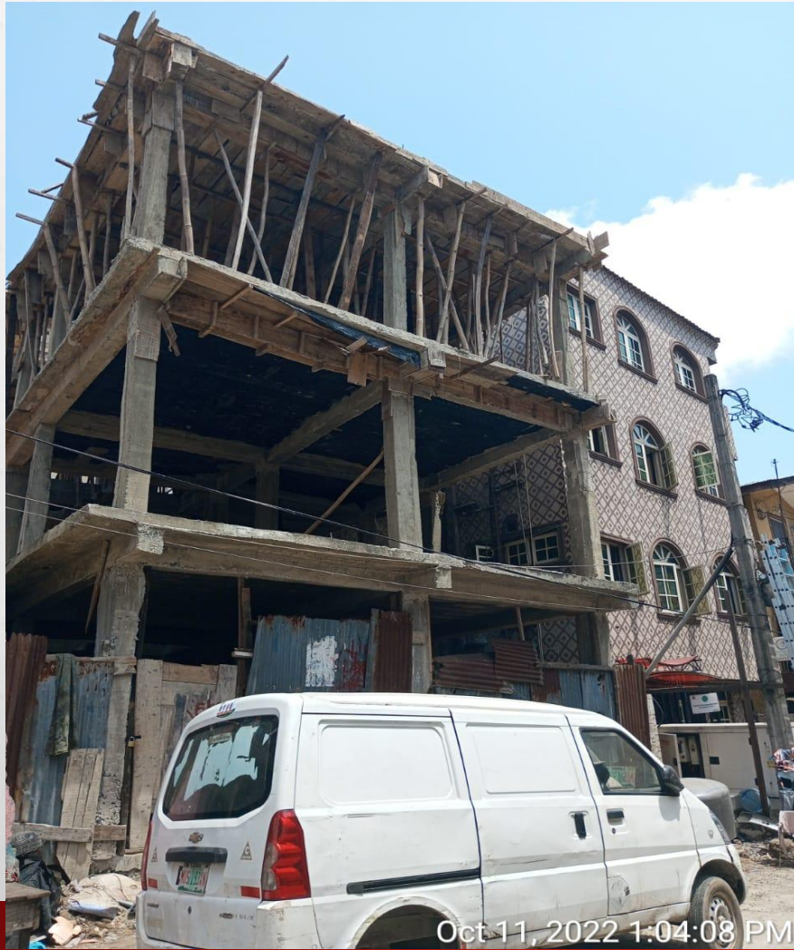
Location: BESIDE 28 ELEGBATA STREET, LAGOS ISLAND. Stage: THIRD FLOOR SLAB
