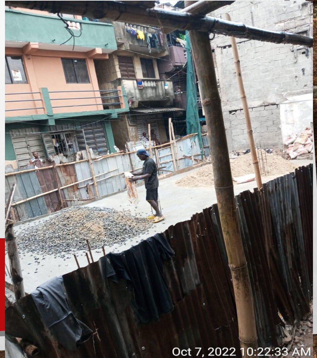
Location: 6 OKITI LANE LAGOS ISLAND Stage: GROUND FLOOR SLAB
