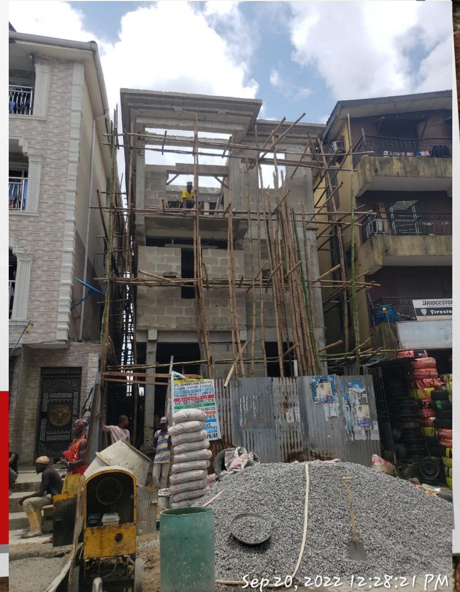
Location: 25, Foresythe Street, Lagos Island, Lagos. STAGE: ROOF PARAPHET
