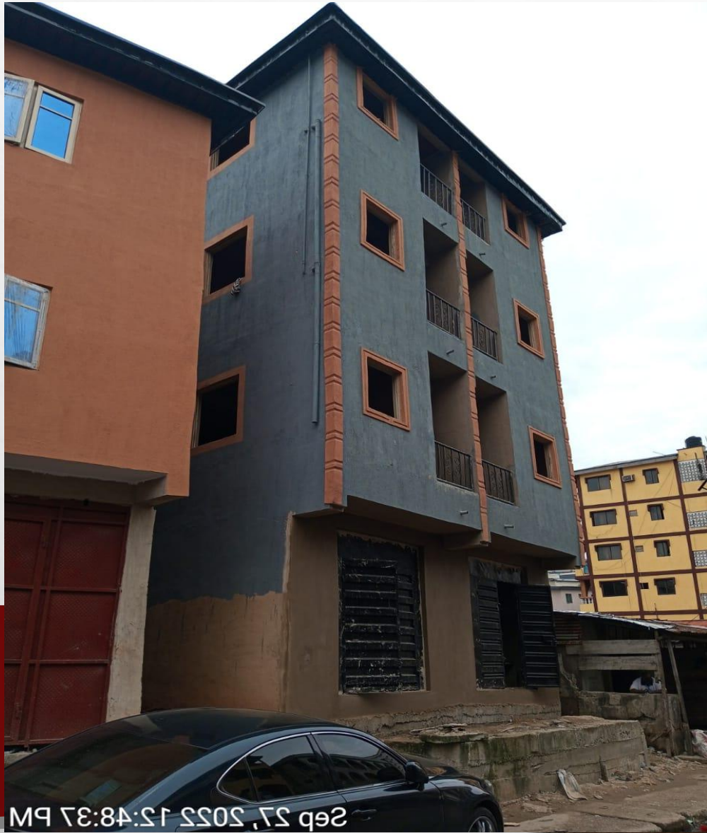
Location: ALONG BINUYO STREET Stage: FINISHES
