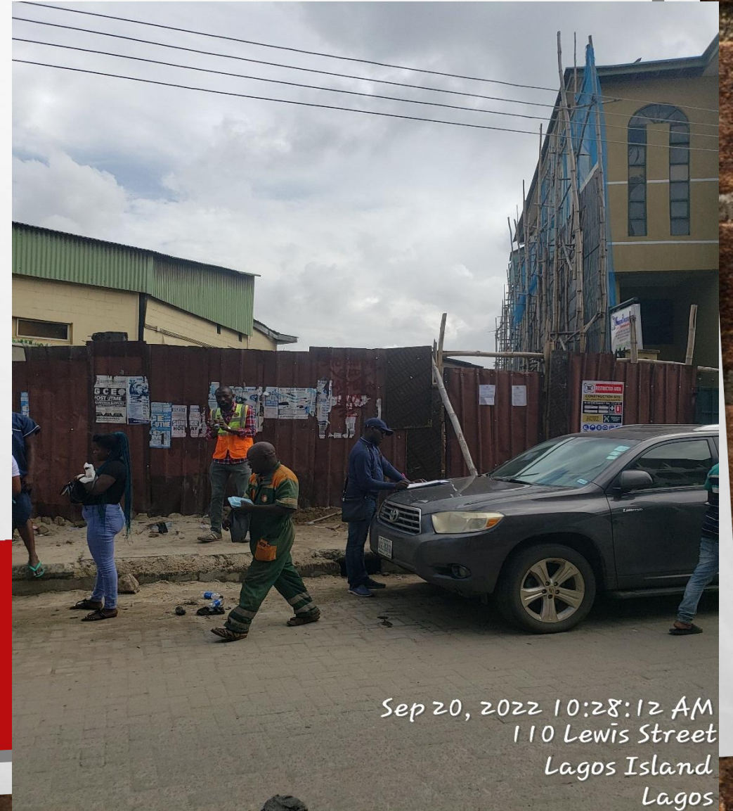
Location: 99A, Lewis Street, Lagos Island, Lagos. STAGE: RAFT FOUNDATION
