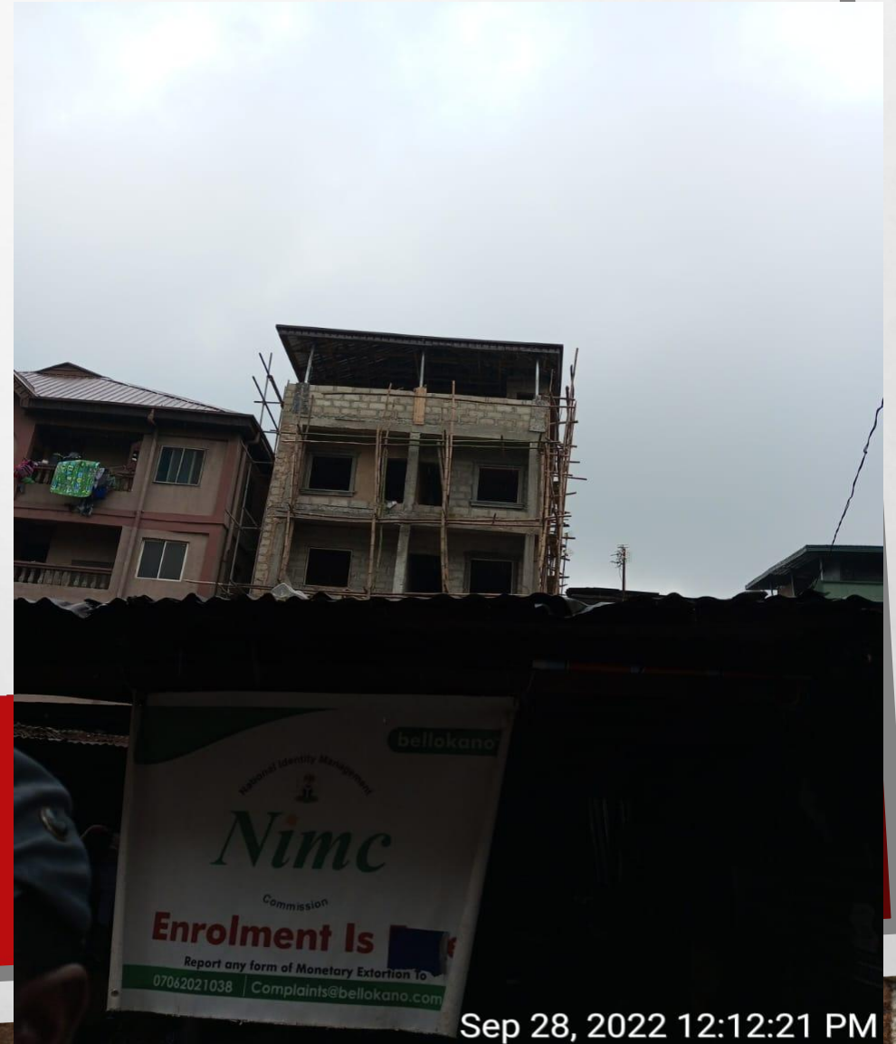
Location: 11, OJU OLOBUN CLOSE Stage: ROOFED
