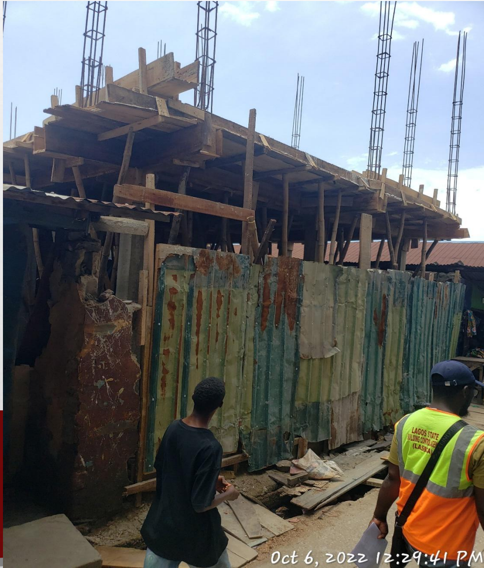
Location: 11, Kingsway Street, Lagos Island, Lagos. STAGE: FIRST SUSPENDED FLOOR SLAB
