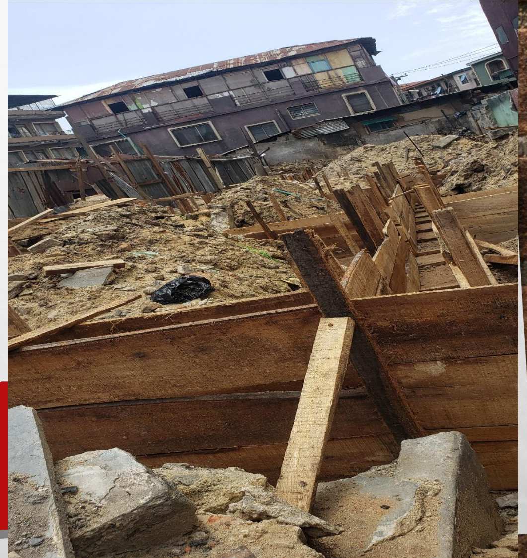
Location: 2, Osho Street, Lagos Island, Lagos. STAGE: RAFT FOUNDATION TRENCHES
