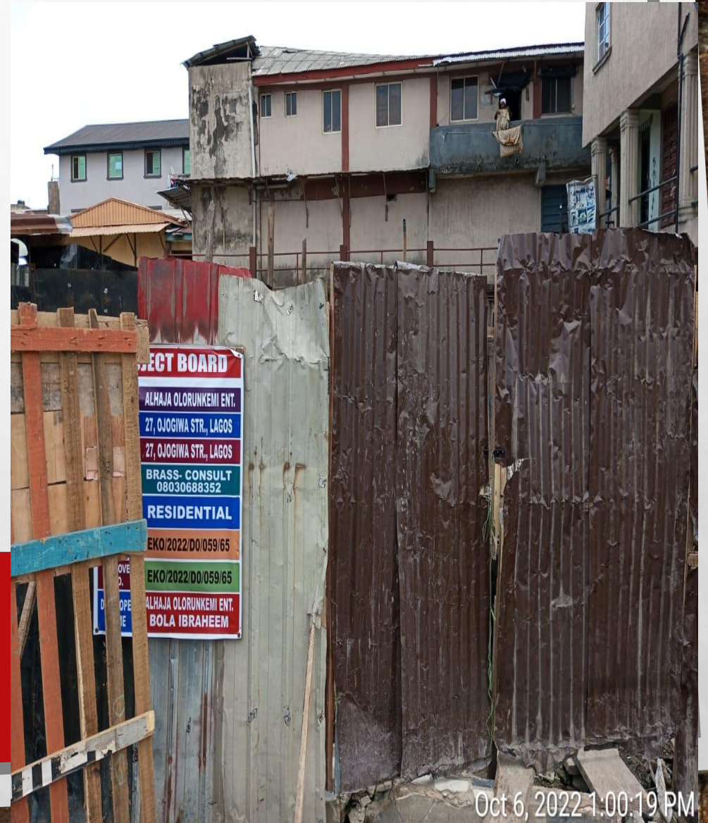
Location: 27 OJO GIWA STREET LAGOS ISLAND Stage: FOUNDATION ONGOING
