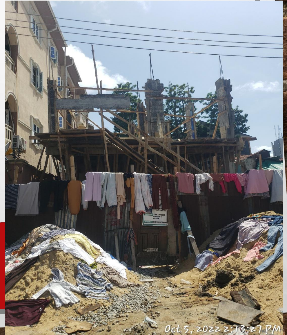
Location: 54, Foresythe Street, Lagos Island, Lagos. STAGE: FIRST FLOOR COLUMN
