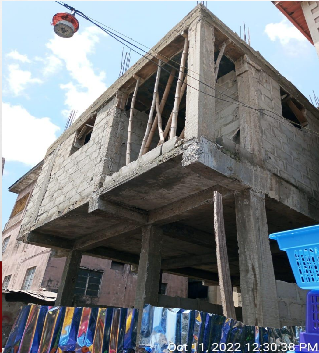
Location: ALONG ALAKORO STREET LAGOS ISLAND Stage: SECOND SUSPENDED FLOOR SLAB
