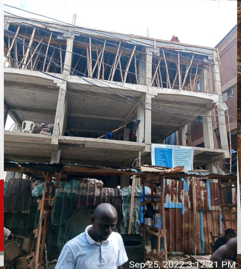
Location: 20 IDI-OLUWO STREET LAGOS ISLAND. Stage: ONGOING AT FOURTH FLOOR SLAB
