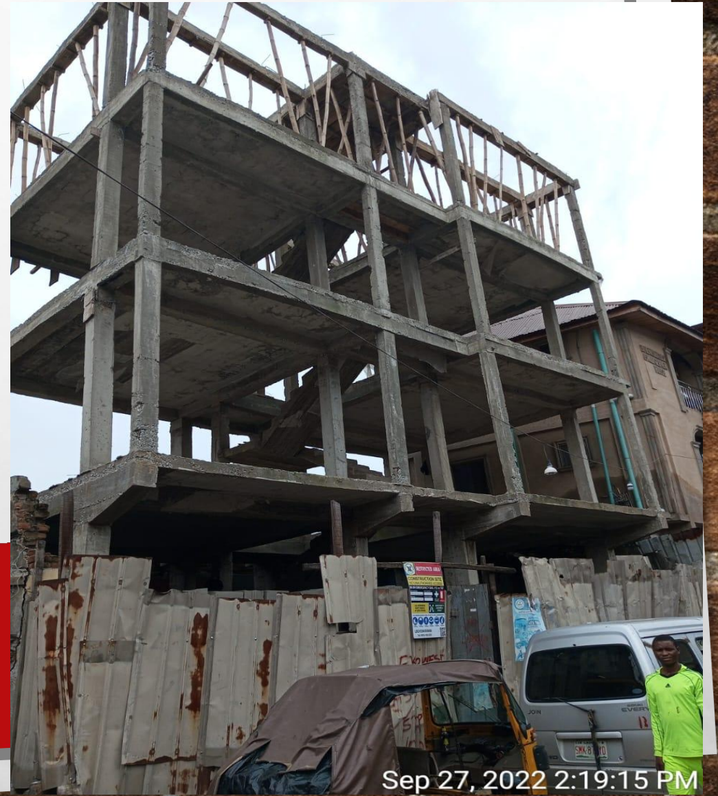
Location: 16, PALM CHURCH STREET Stage: ROOF BEAM
