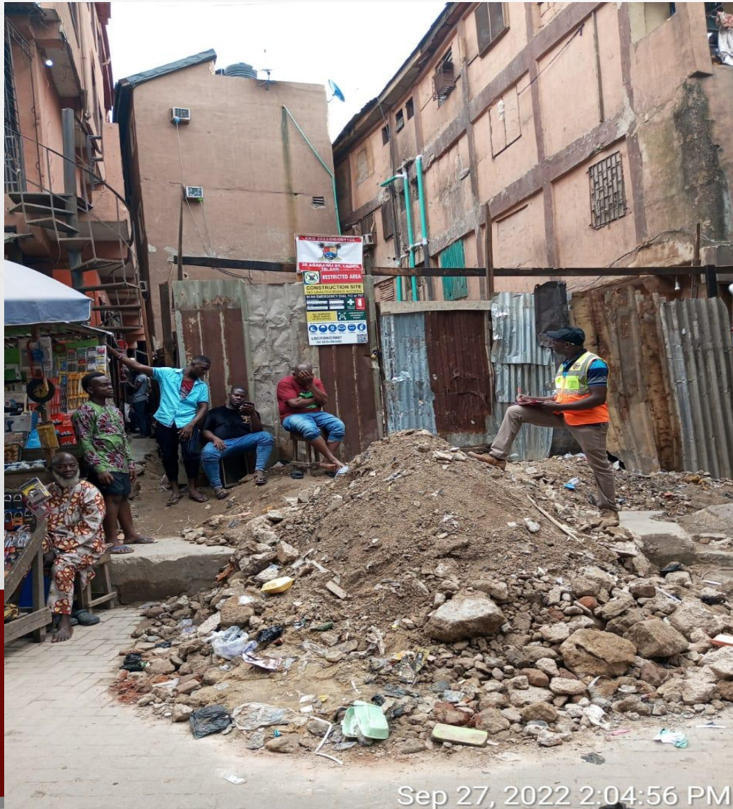
Location: 26 AGARAWU STREET LAGOS ISLAND Stage: FOUNDATION ONGOING
