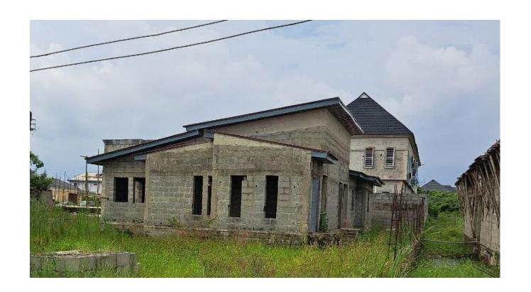
STAGE OF WORK: FIRST FLOOR SLAB, ABANDONED
