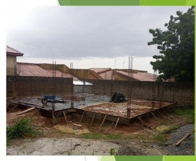
SETTING OUT --- EXCAVATION – BLINDING --- REBAR PLACEMENT –CASTING FOR PAD FOUNDATION
