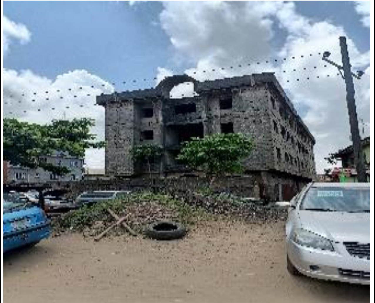
Property Along Ishashi Road, opposite Dickem Farm Close, Ishashi
