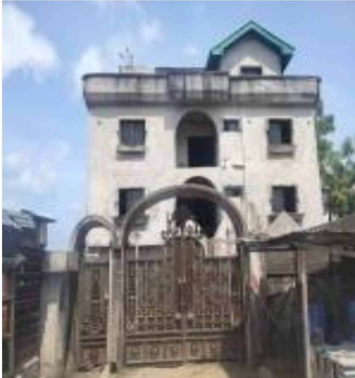
Along Etegbin road, Oto-Awori.
