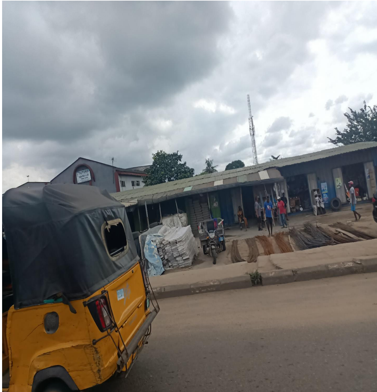
Along Lasu-iba Expressway, Agboroko Busstop, Iba
