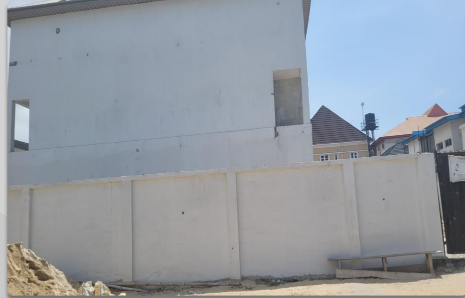
2 FLOORS ALONG HAKEEM DICKSON. APPROVAL STATUS- NOT ASCERTAINED NO OF FLOORS- 2 FLOORS
