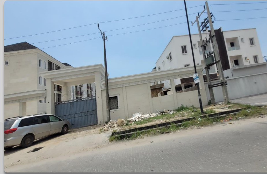
ALONG WHITE SANDS AVENUE, LEKKI 1 APPROVAL STATUS- NOT ASCERTAINED NO OF FLOORS- 4 FLOORS, 4 BLOCKS
