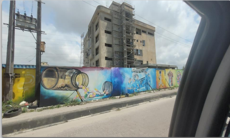
5+ PENT STRUCTURE ALONG T.F KUBOYE LEKKI 1 (DCB 25815 ET) APPROVAL STATUS- APPROVED STAGE CERTIFICATION - ONGOING NO OF FLOORS- 5 + PENT FLOORS
