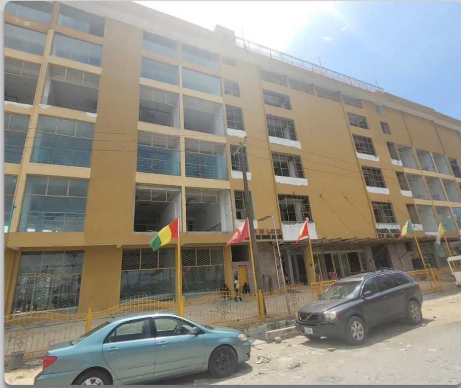
BANEX BUILDING AKIOGUN ROAD LEKKI 1 APPROVAL STATUS- APPROVED STAGE CERTIFICATION - ONGOING NO OF FLOORS- 6 FLOORS
