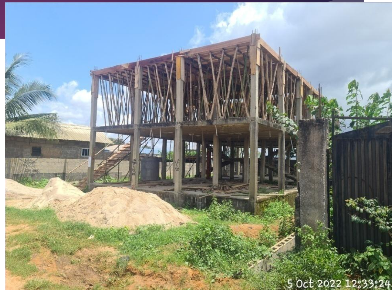
ALONG LEKKI-EPE EXPRESSWAY, BY T-JUNCTION, EPE. STAGE OF WORK: THIRD FLOOR SLAB FORMWORK IN PROGRESS
