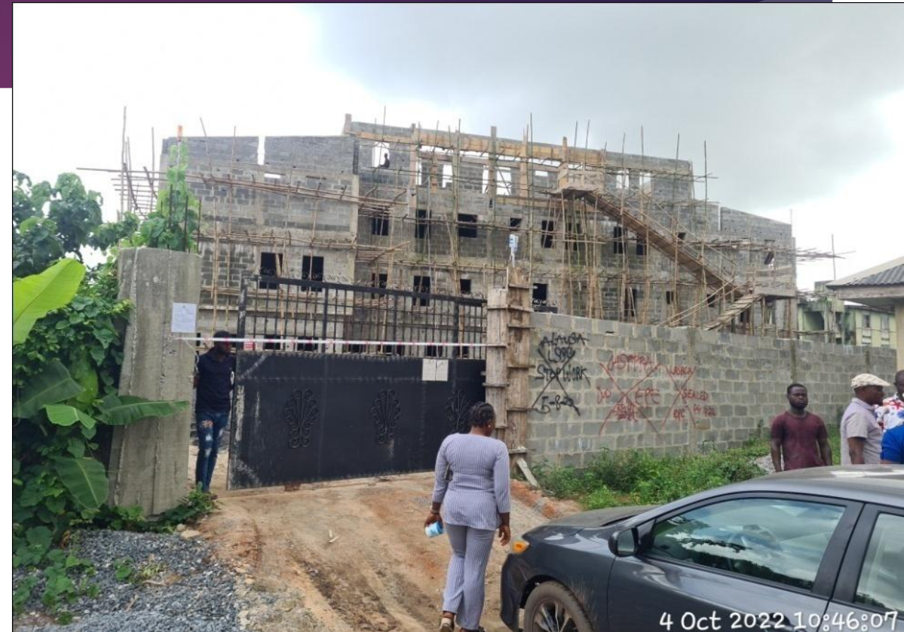
PROPERTY OFF EPE-IJEBU ODE ROAD, OPPOSITE NIGERIA LAMP INDUSTRY, ODOMOLA, EPE. STAGE OF WORK: 4TH FLOOR LINTEL LEVEL
