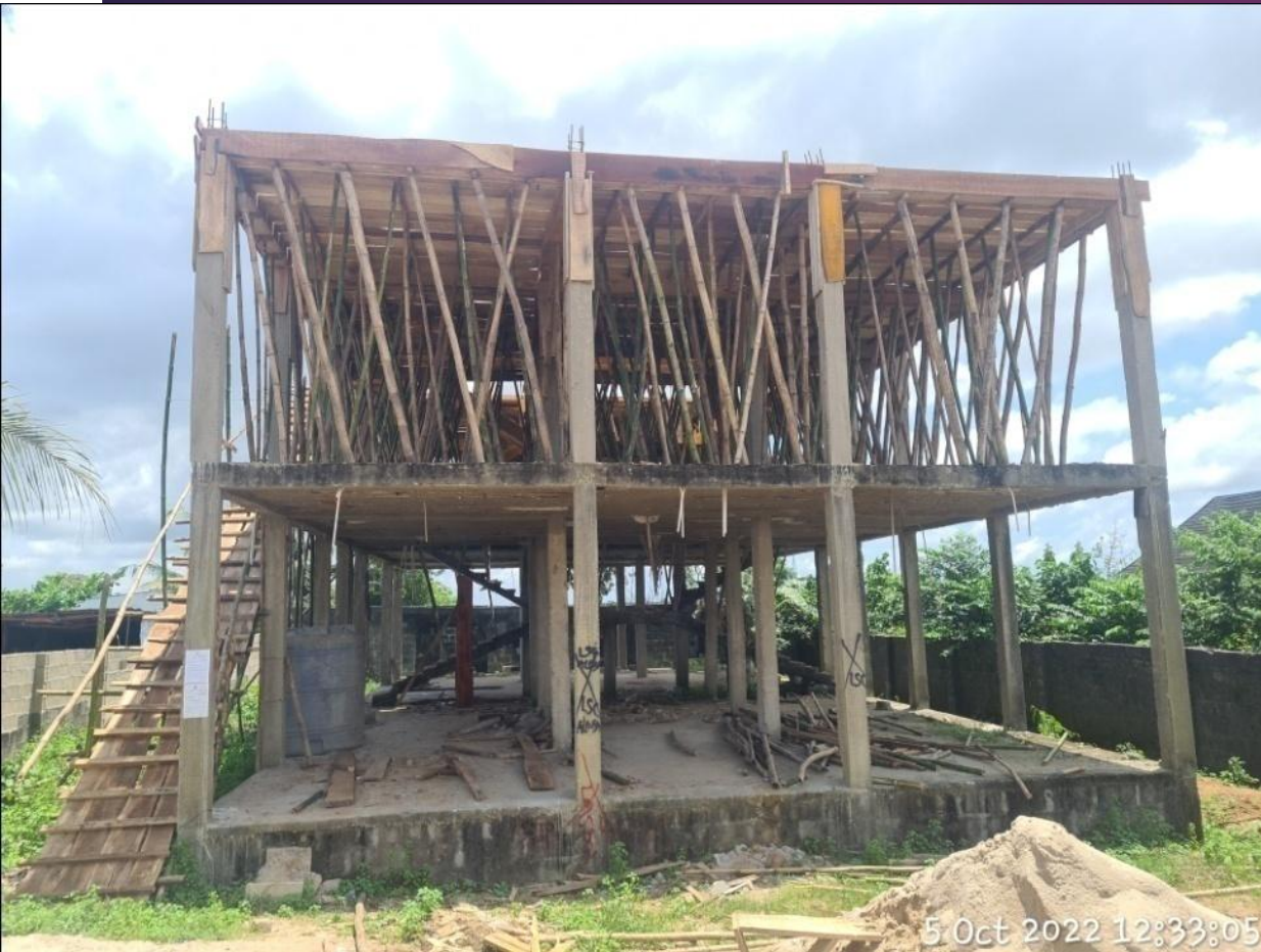
ALONG LEKKI-EPE EXPRESSWAY, BY T-JUNCTION, EPE. STAGE OF WORK: THIRD FLOOR SLAB FORMWORK IN PROGRESS
