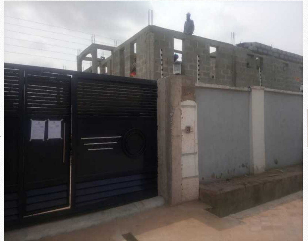
PROPERTY BESIDE NO 10, OREMEJI STREET, AGODO, EGBE-IDIMU, LAGOS
