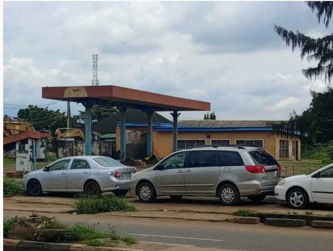
PETROL FILLING STATION ALONG IDIMU-IKOTUN ROAD, BESIDE ENILOBO CLOSE, EGBE-IDIMU, LAGOS
