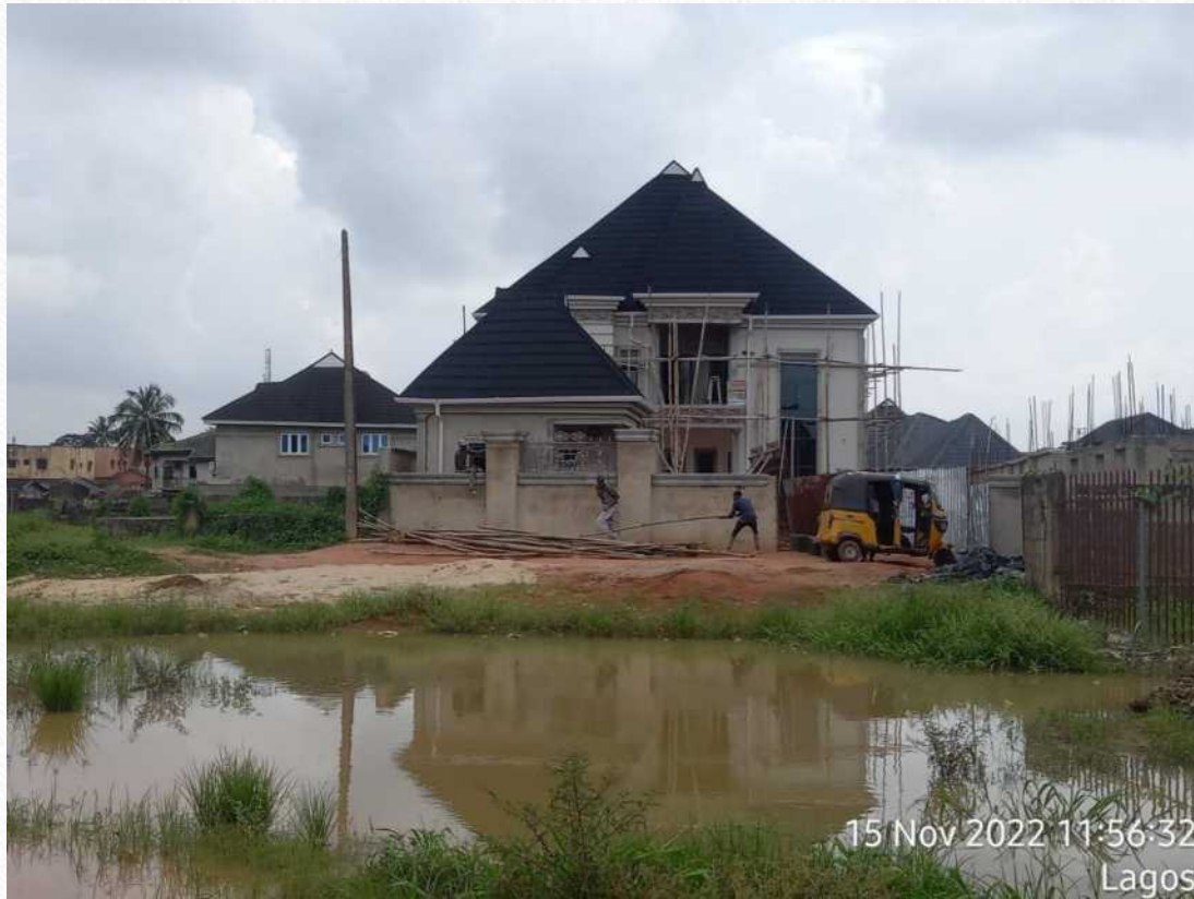
PROPERTY ALONG PIPELINE ROAD, LASU-SIHERI, EGBE-IDIMU, LAGOS
