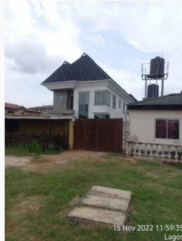
PROPERTY ALONG PIPELINE ROAD, LASU-SIHERI, EGBE-IDIMU, LAGOS
