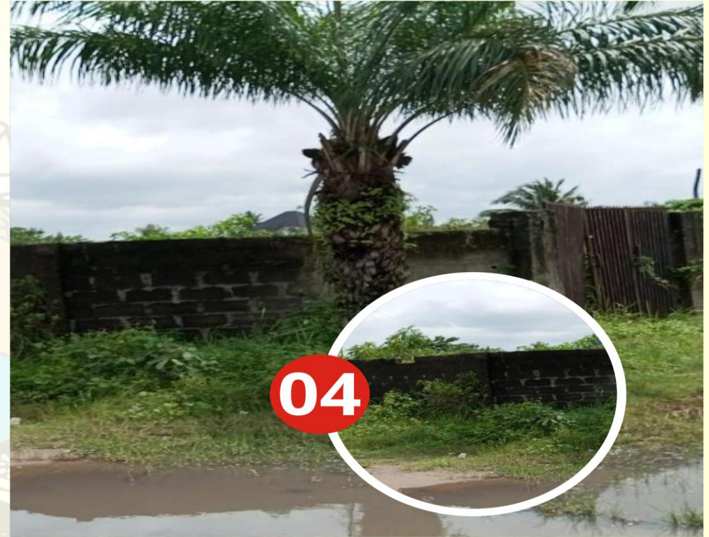
ALONG OKE-OWO STREET OFF ITOGA ROAD, BADAGRY DATE CAPTURED: 20/09/2022
