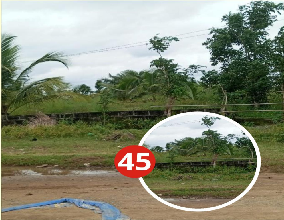
ALONG ASCON ROAD, IDALE, BADAGRY DATE CAPTURED: 27/09/2022
