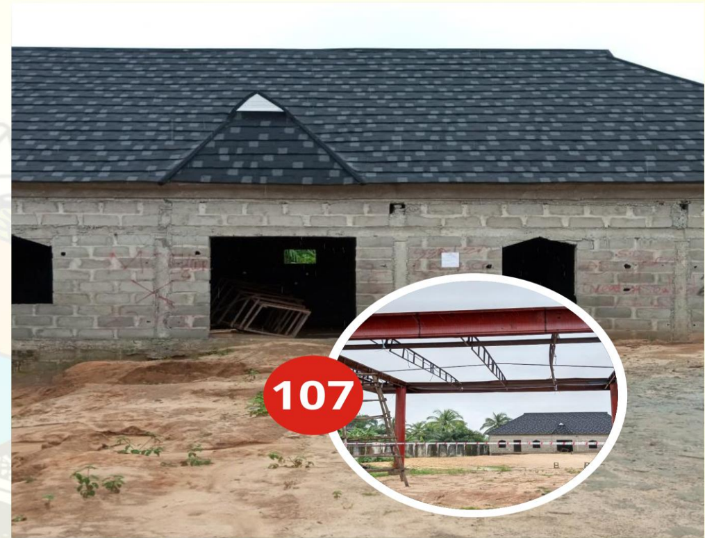
BESIDES FEDERAL ROAD SAFETY OFFICE, AJARA TOPA, BADAGRY DATE CAPTURED:22/09/2022
