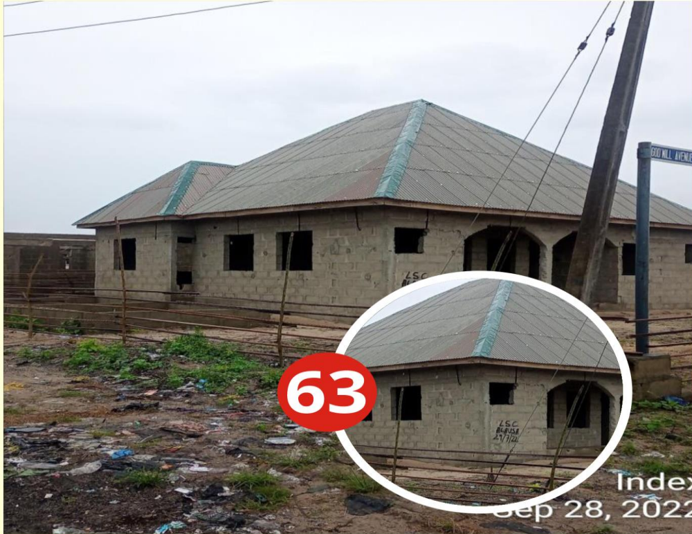
UNDER CONSTRUCTION AT GOFAMINT STREET POVITA, BADAGRY DATE CAPTURED: 28/09/2022
