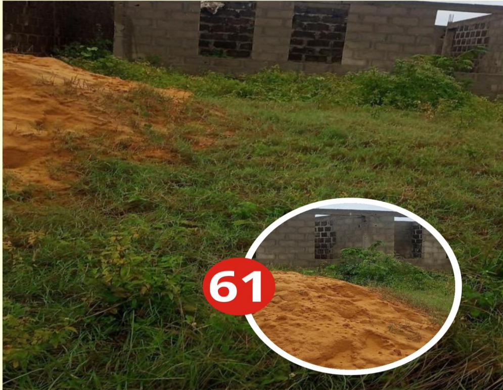
ALONG OKE-OWO STREET OFF ITOGA ROAD, BADAGRY DATE CAPTURED: 20/09/2022
