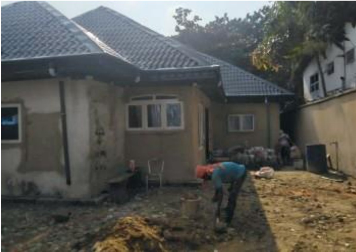
The property beside NO 7B, Oduduwa road, GRA, Apapa.
