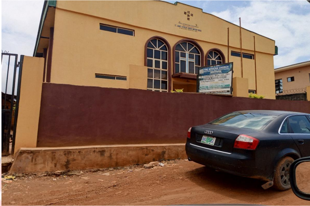
52. ST JAMES AFRICAN CHURCH AT 24 BAALE STREET
