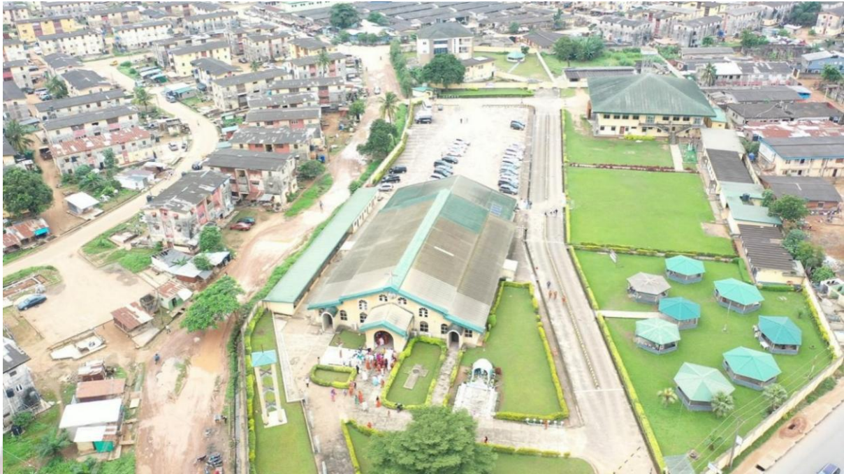
40. ST FERDINARD CATHOLIC CHURCH AT 215 SECTOR 6 ROAD, ABESAN ESTATE
