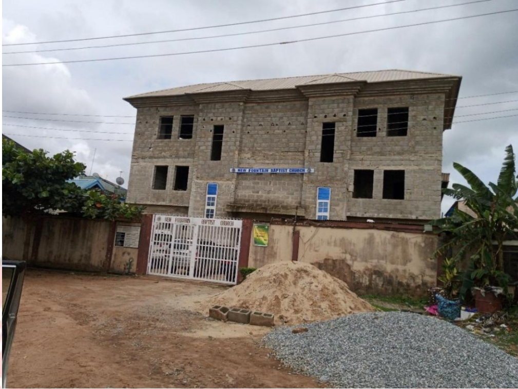
112. NEW FOUNTAIN BAPTIST CHURCH 12 TH ROAD, 1 ST AVENUE, GOWON ESTATE EGBEDA
