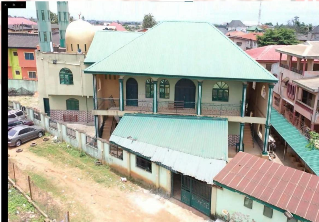
7. ANSAR UD DEEN SOCIETY MOSQUE (IPAJA) AT GATE BUS STOP
