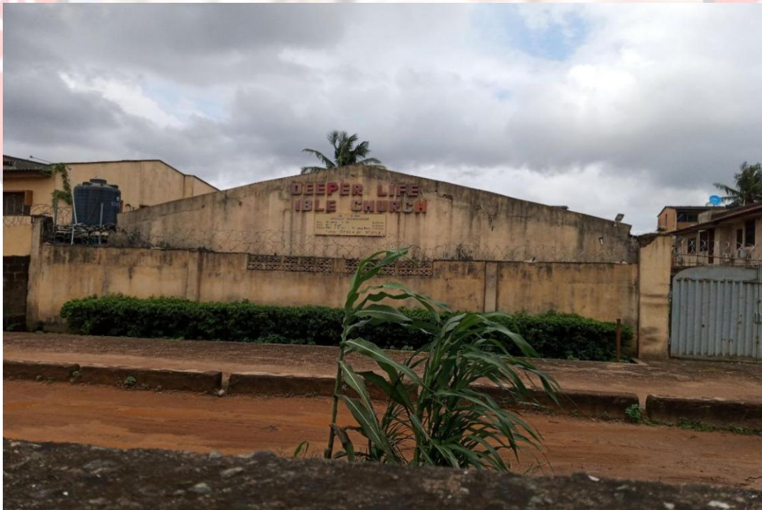
77. DEEPER BIBLE CHURCH AT 1 ST AVENUE 41 ROAD GOWON ESTATE EGBEDA
