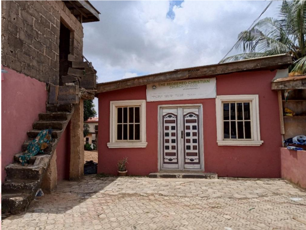
102. THE REDEEMED CHRISTIAN CHURCH OF GOD ALONG OLANREWAJU ARIYIBI STREET ODO ERAN BUS STOP, ABULE ONILU ALONG ISHERI EXPRESS WAY
