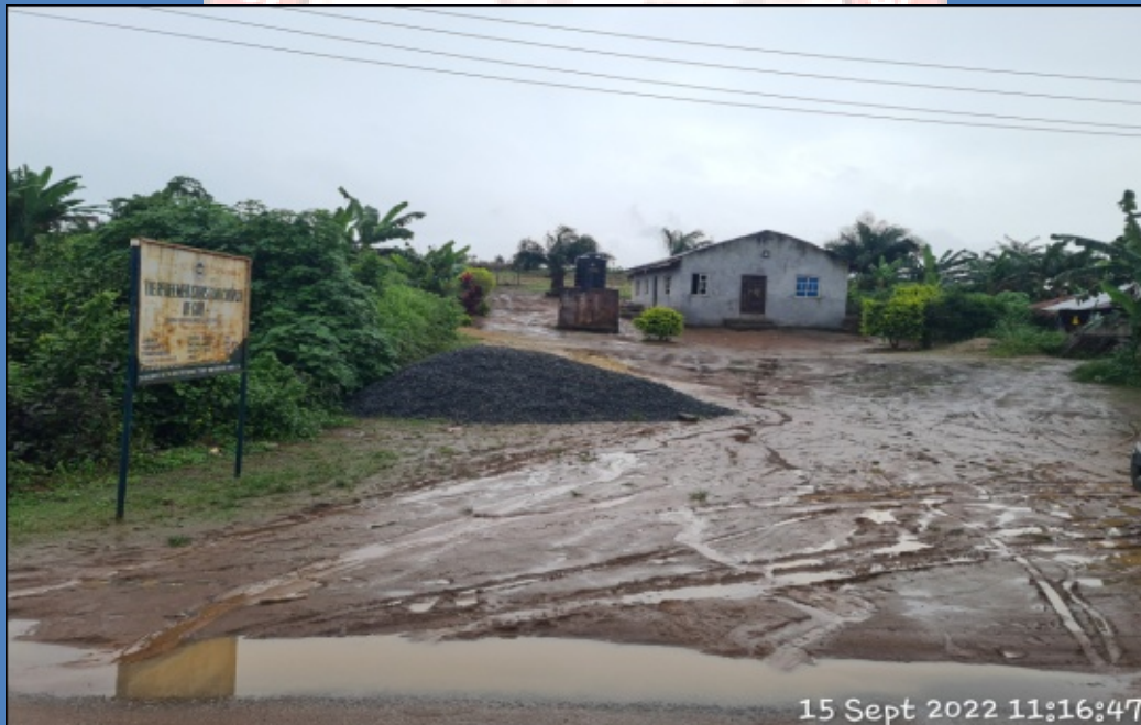
NAME: THE REDEEMED CHRISTAIN CHURCH OF GOD ADDRESS: ERERUFU, AGBOWA, IKOSI EJIRIN LCDA, EPE DEFECTS: NIL
