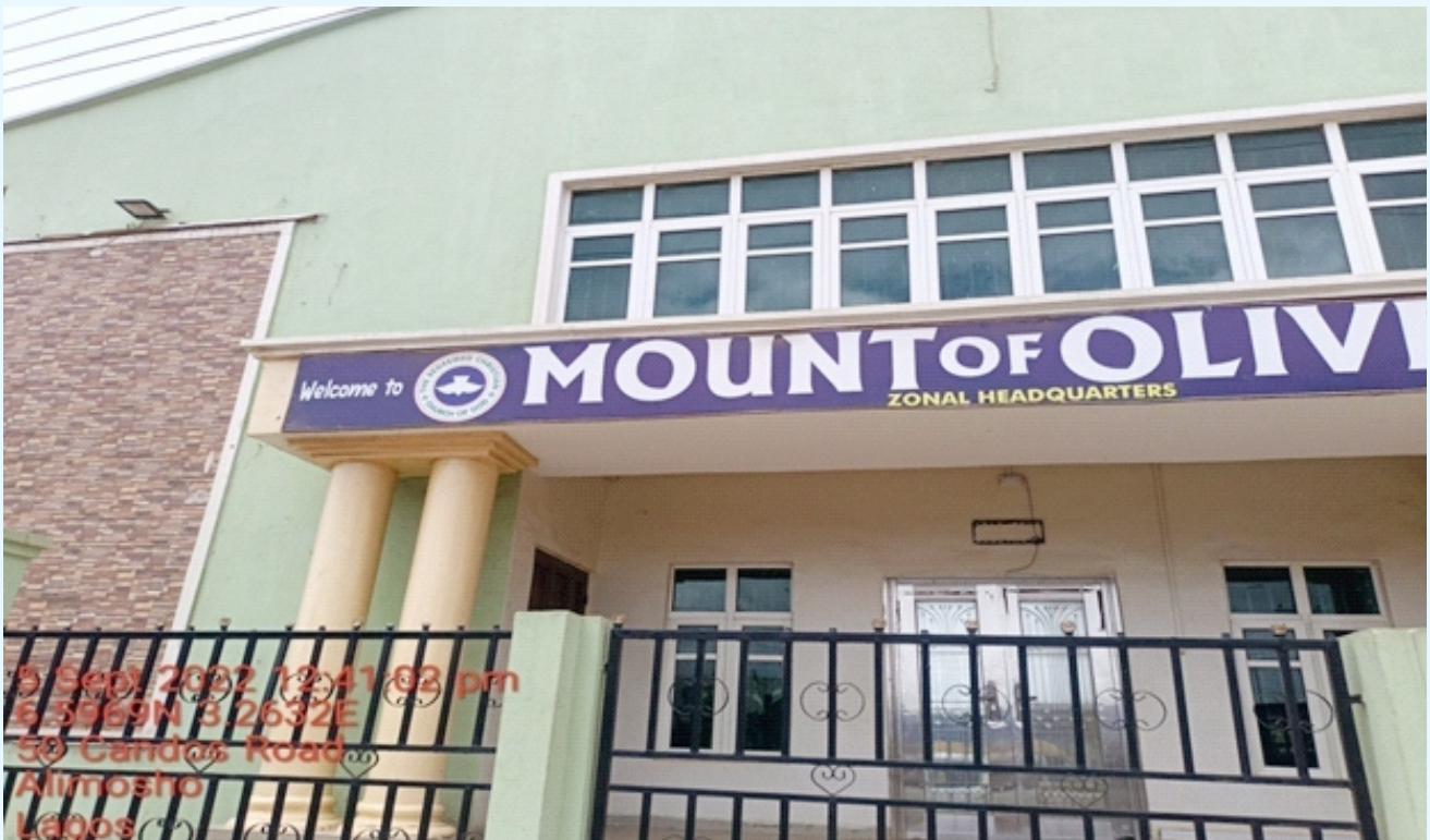
THE REDEEM CHRISTIAN CHURCH OF GOD LP 12, 36 CANDOS ROAD, BARUWA IPAJA. (2-FLOORS)
