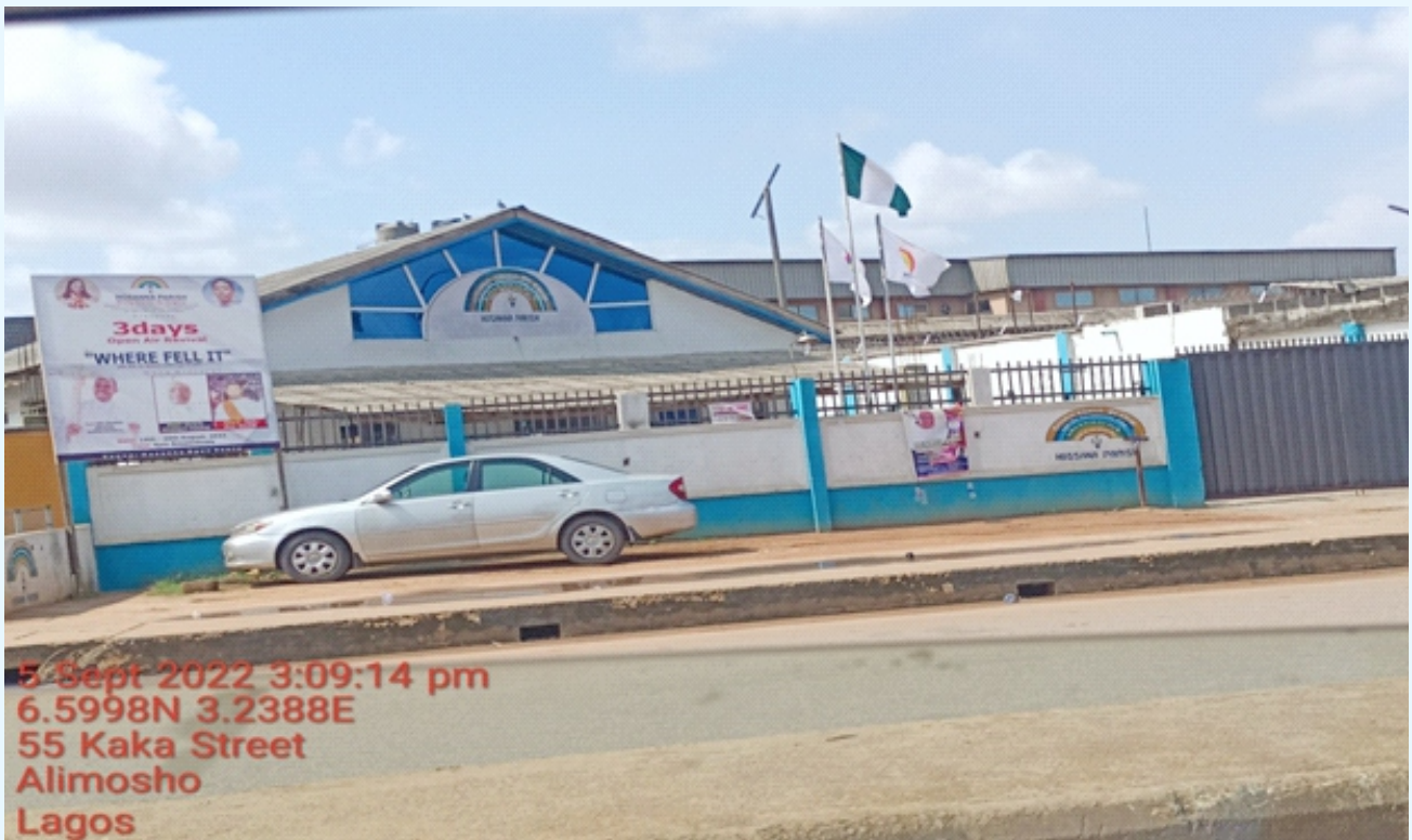
HOSANA PARISH ALONG AYOBO ISEFUN NEW EXPRESS ROAD, OPPOSITE AYOBO MAIN MARKET, AYOBO LAGOS. (BUNGALOW).
