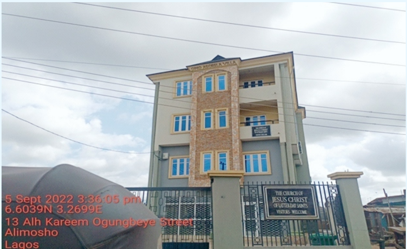
CHURCH OF JESUS CHRIST, OMOASHORELA BUILDING, BARUWA BUS-STOP, IPAJA (4-Floors)
