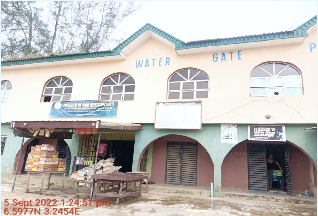
CHURCH OF GOD MISSION INT'L, 3 KASALI STREET, OFF ASHIPA ROAD, AMULE BUS-STOP, AYOBO IPAJA, LAGOS. (2-FLOORS).
