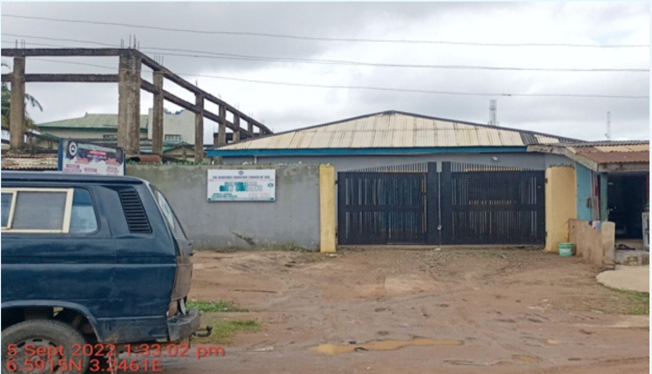
THE REDEEMED CHRISTIAN CHURCH OF GOD, REHOBOTH PARISH, LP 24, 81 ASHIPA ROAD, AMULE, AYOBO. 2-FLOORS
