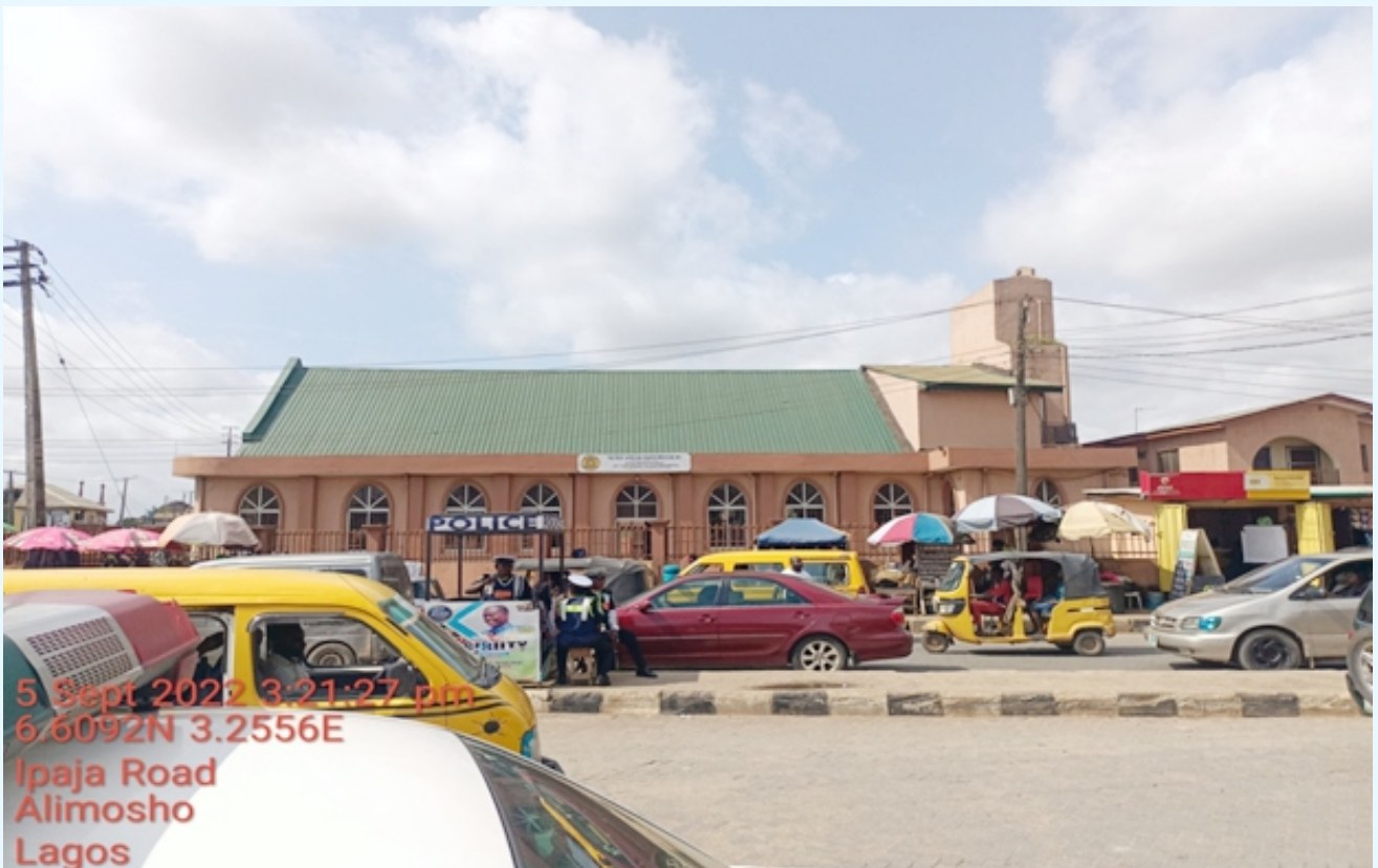
THE FIRST AFRICAN CHURCH MISSION INC, 1 COMMAND ROAD, IPAJA, LAGOS. (BUNGALOW).
