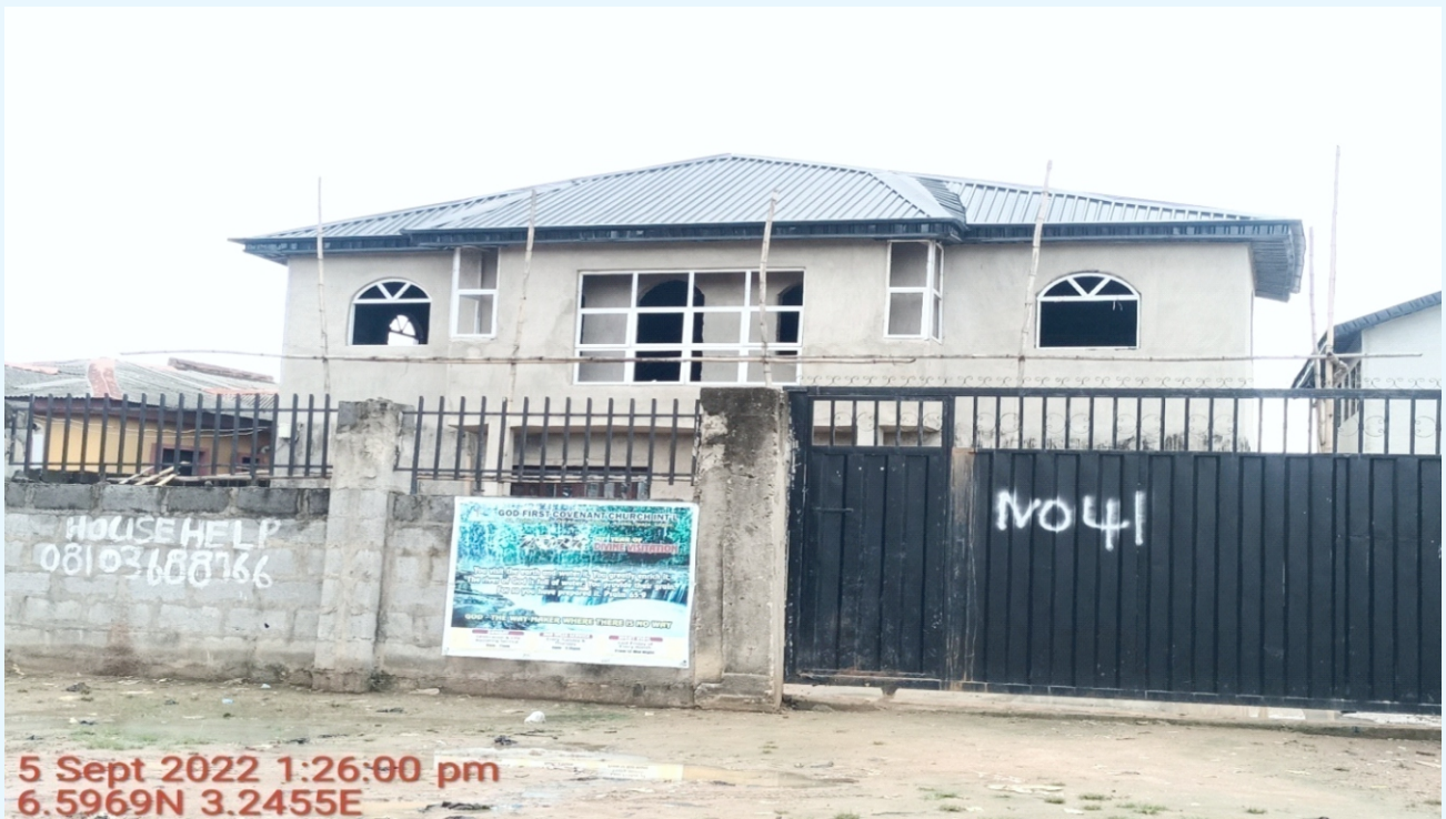
GOD FIRST COVENANT CHURCH INT'L, 41 ASHIPA ROOF, OFF AMULE BUS-STOP, AYOBO, LAGOS. (2-FLOORS).
