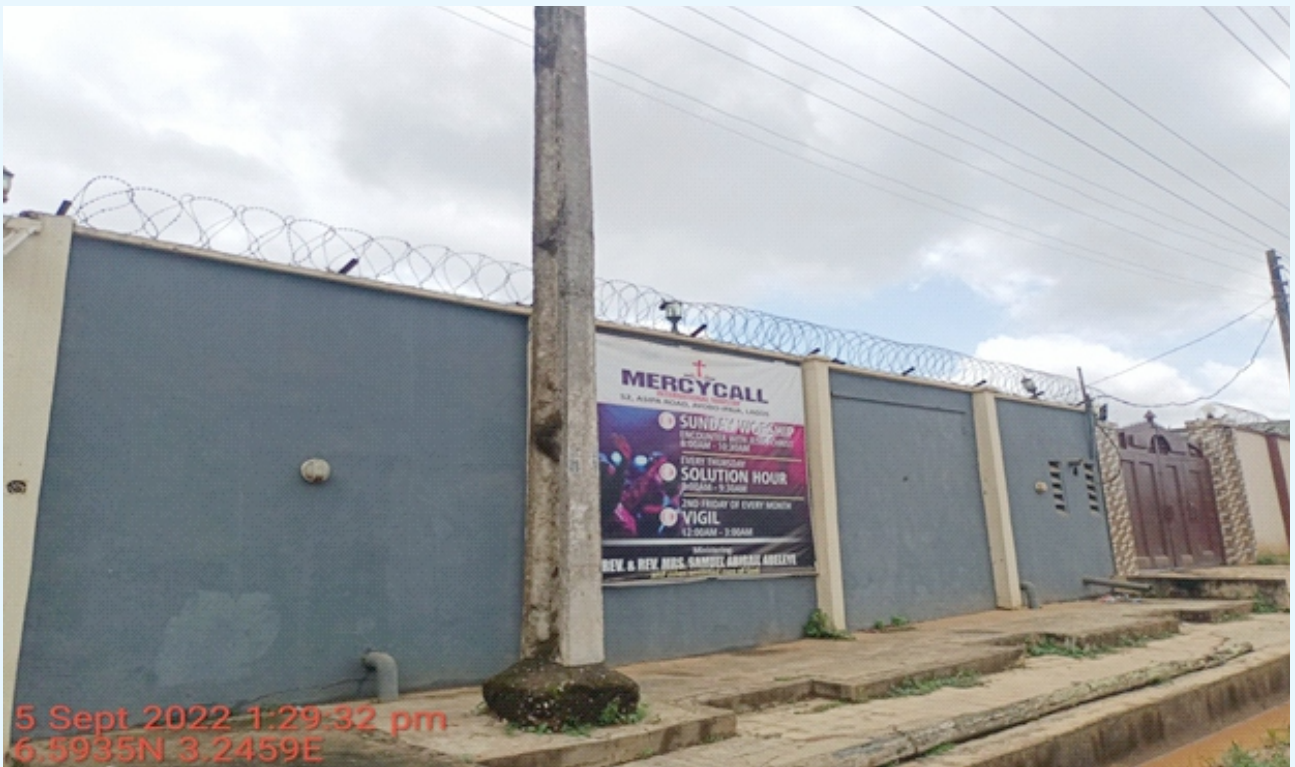
MERCY CALL INTERNATIONAL MINISTRY 52, ASIPA ROAD, AYOBO, LAGOS. (2-FLOORS).
