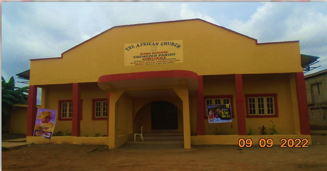
THE AFRICAN CHURCH:- 30 EKORO ROAD, AGBELEKALE, ABULE-EGBA
