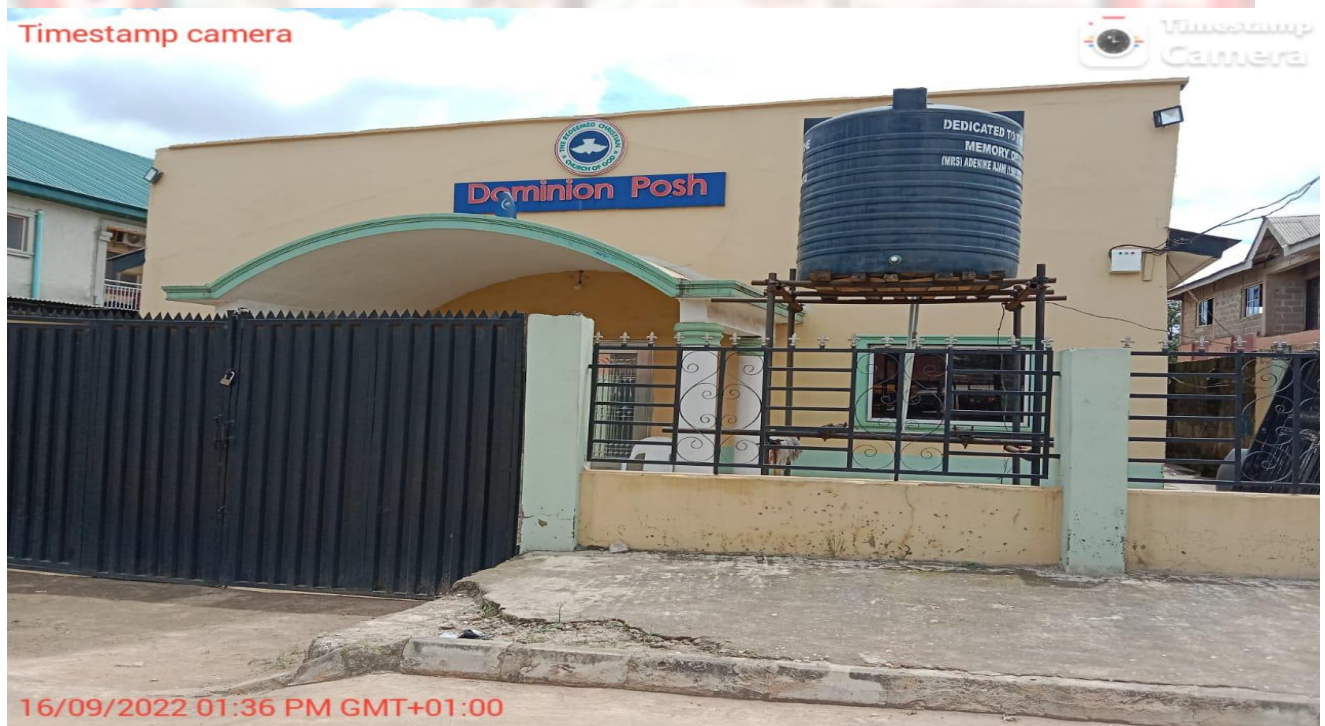
THE REDEEMED CHRISTIAN CHURCH OF GOD (DOMINION POSH):- 33 OLD OTTA ROAD, JOKE-AYO, ALAGBADO
