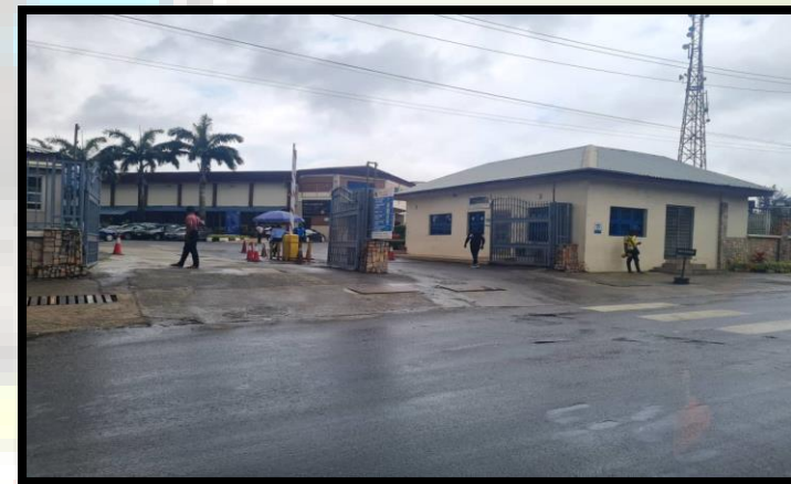
Photograph showing the Subject Site
