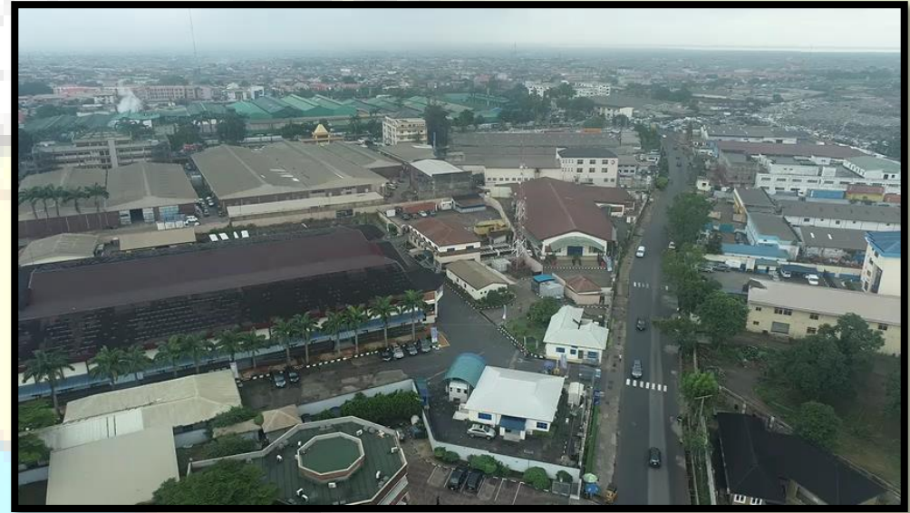
Video coverage of the subject site with the aid of a drone
