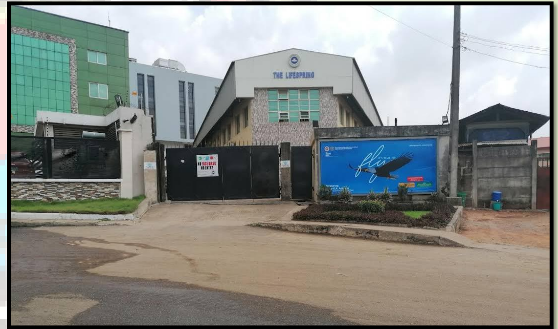
Photograph showing the Subject Site
