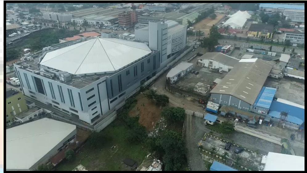
Video coverage of the subject site with the aid of a drone
