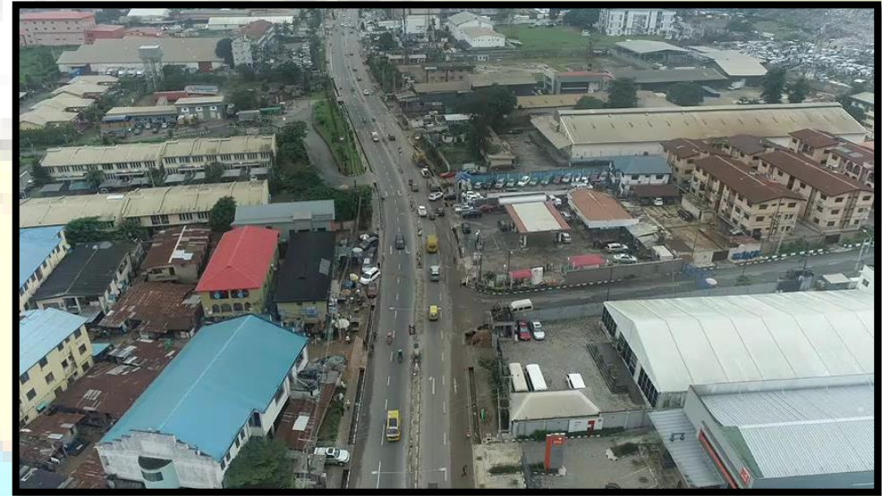
Video coverage of the subject site with the aid of a drone
