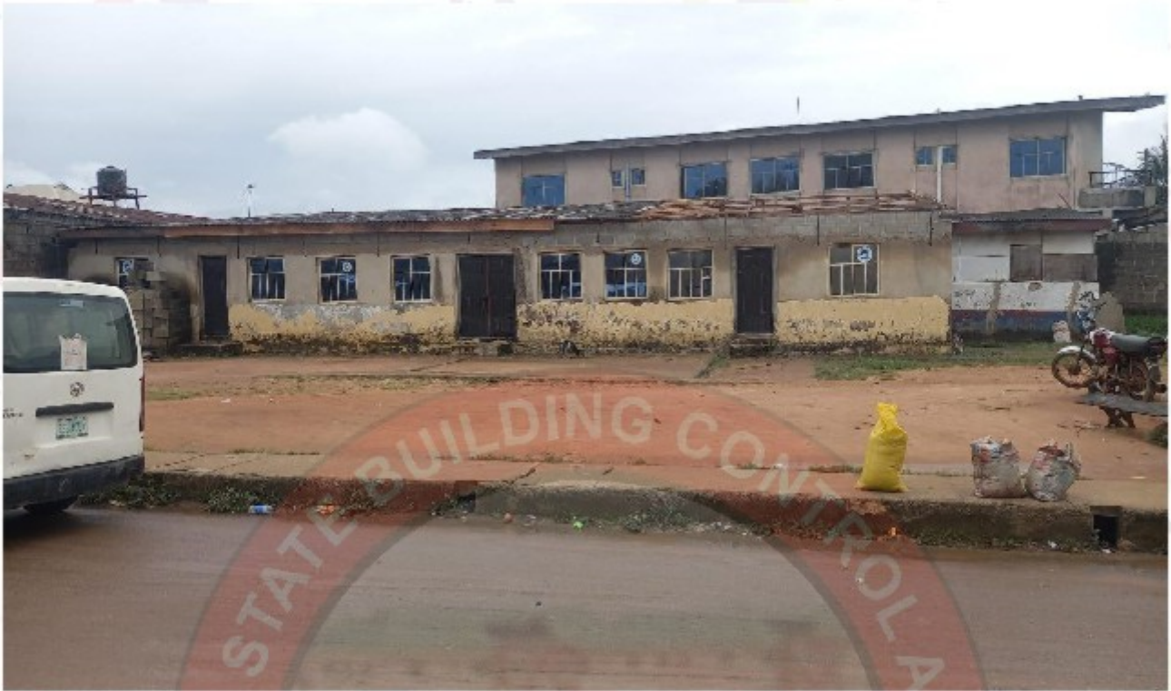
THE REDEEMED CHRISTIAN CHURCH OF GOD, ALONG COMMUNITY ROAD, AGODO, EGBE IDIMU, LAGOS
