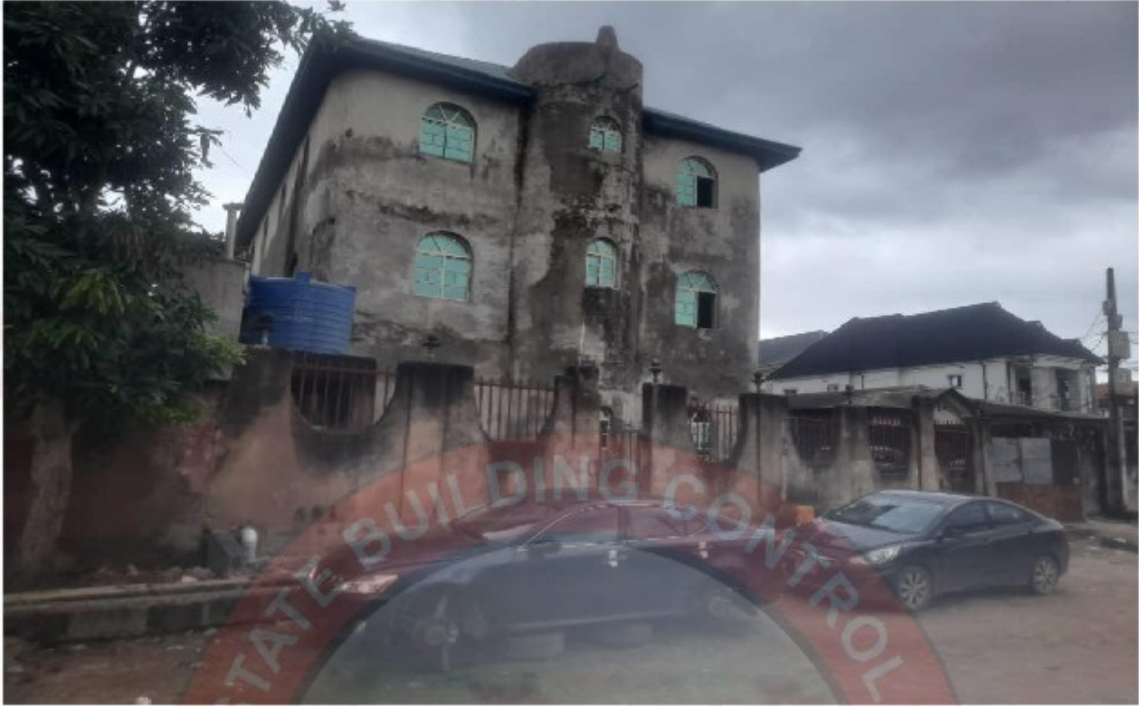
TEMITOPE CENTRAL MOSQUE OPPOSITE GRACE PATHFINDER NURSERY AND PRIMARY SCHOOL, MICHAEL SHOSANYA STREET, OLAJIDE AVENUE, LIASU ROAD, EGBE-IDIMU, LAGOS
