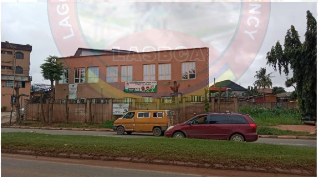
REDEEMED CHRISTIAN CHURCH OF GOD, (TOWER OF PRAISE PARISH) NO 1 KAOMA STREET, OFF LASU IGANDO ROAD, OPPOSITE MICLARA REGENCY HOTEL LAGOS
