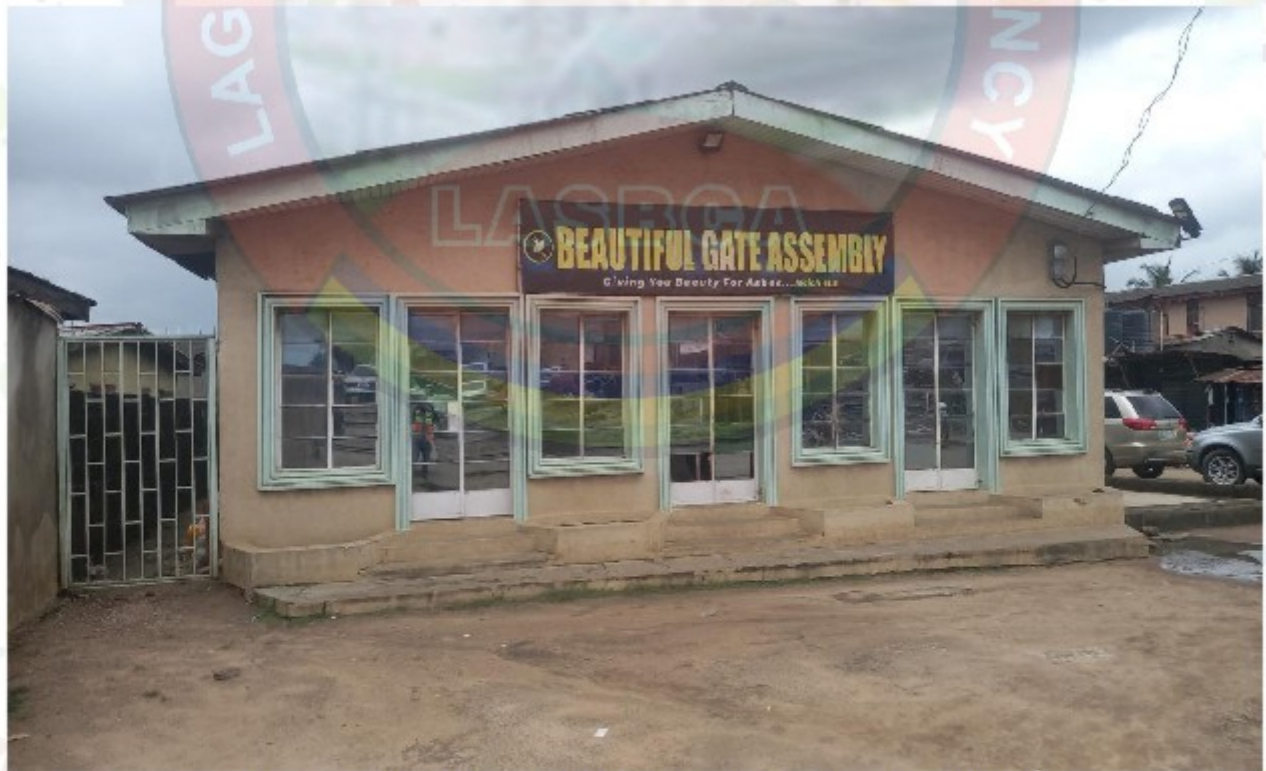
BEAUTIFUL GATE ASSEMBLY, OLADUN ROAD , EGBE IDIMU LAGOS
