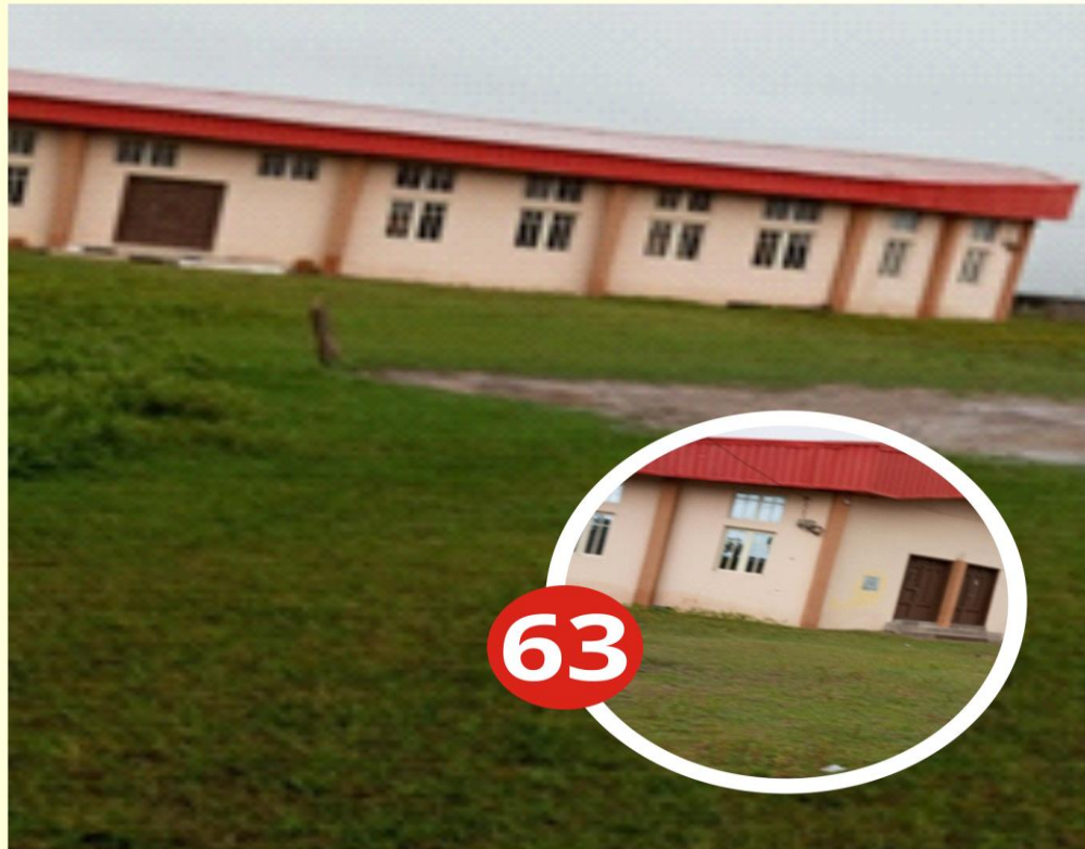
METHODIST CHURCH OF NIGERIA ADDRESS: REV. CADMUS AGOSU STREET DATE CAPTURED:22/09/2022
