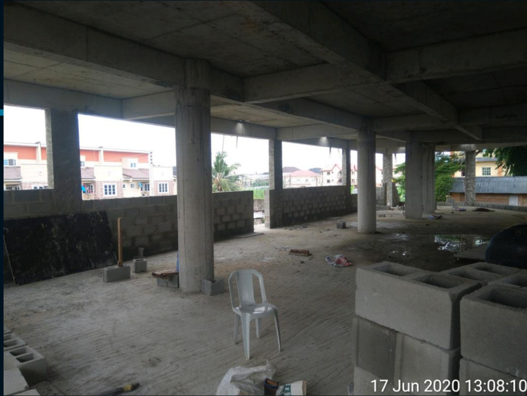
Structural framework with blockwork ongoing
