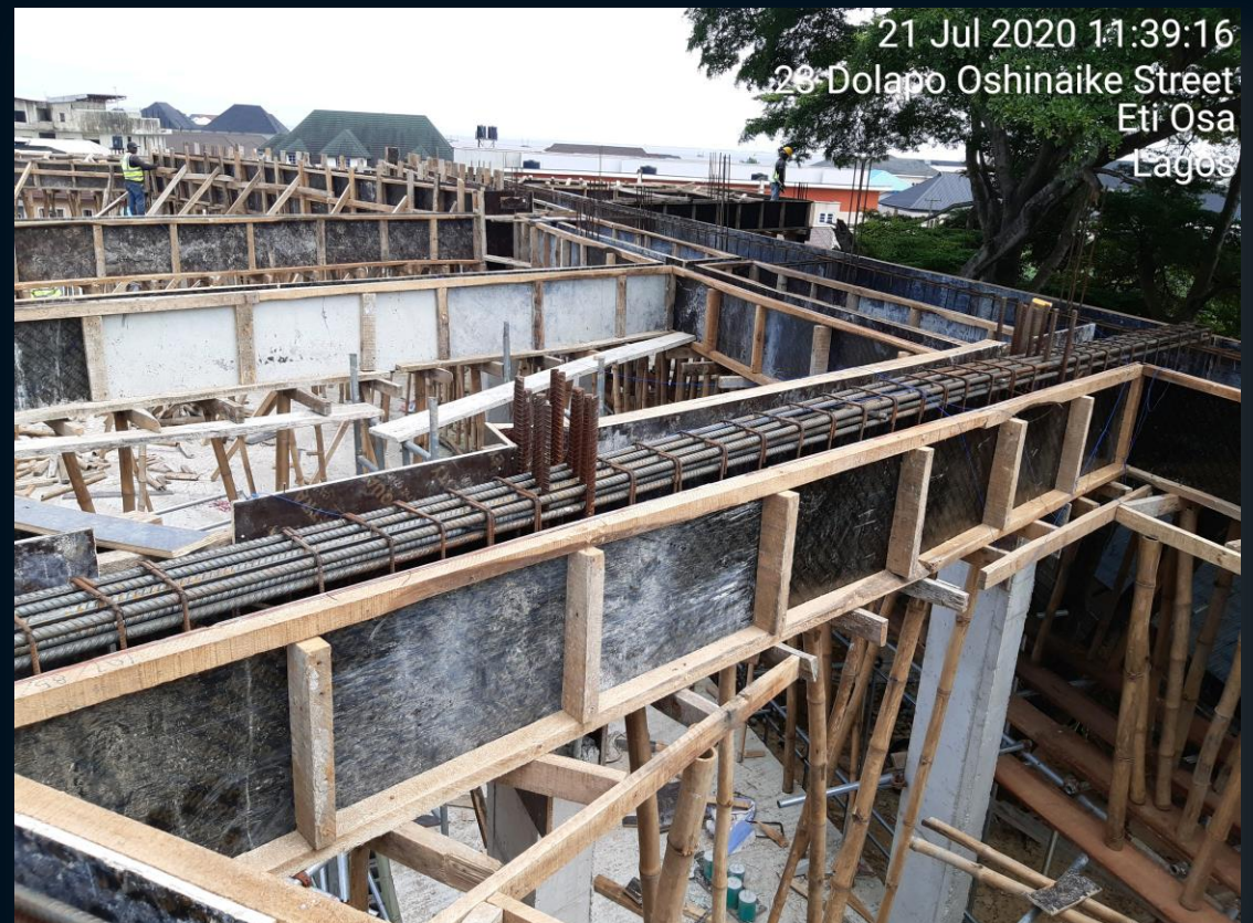
Roof Beams/Gutter Reinforcement placement
