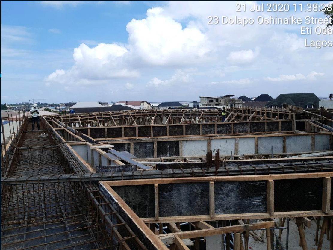
Roof Beams/Gutter Reinforcement placement
