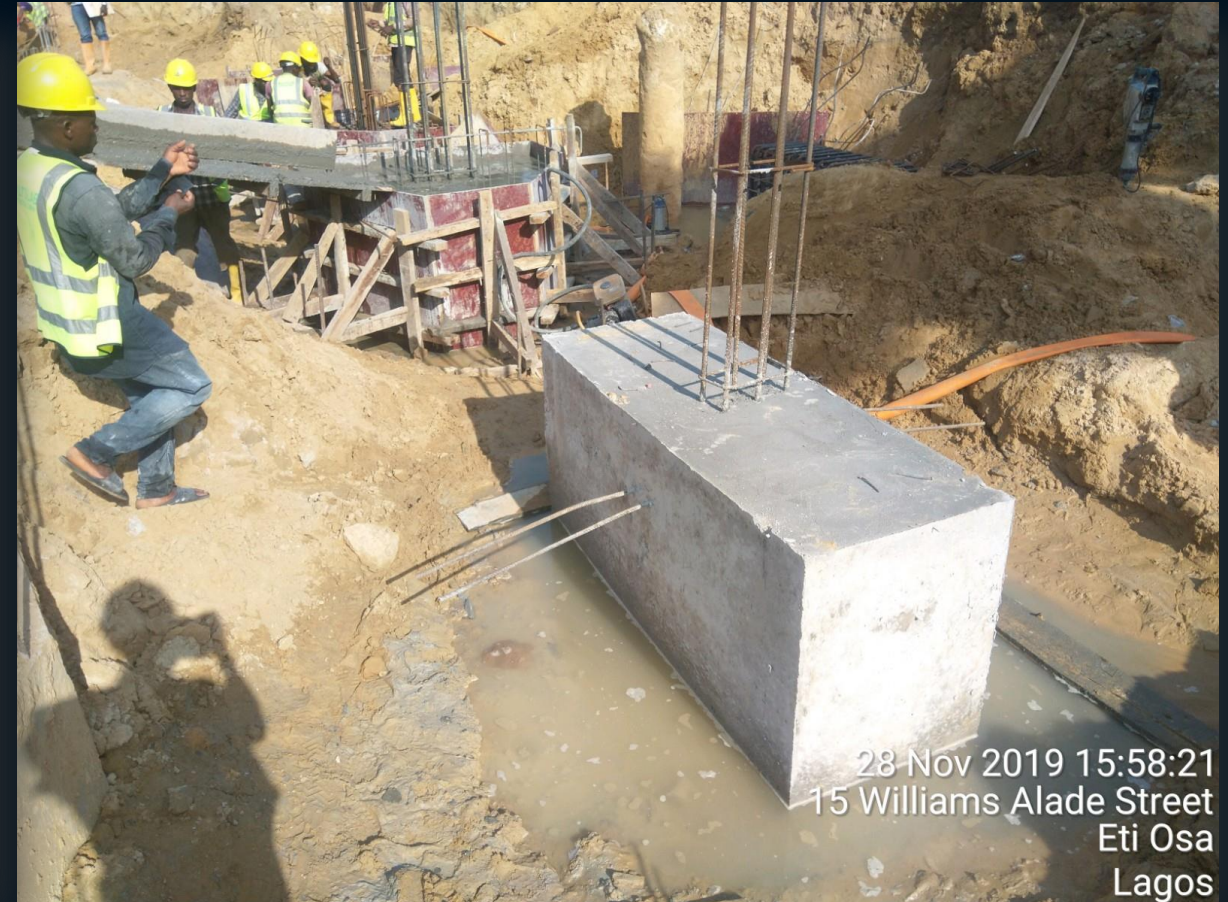
Construction of pile cap
