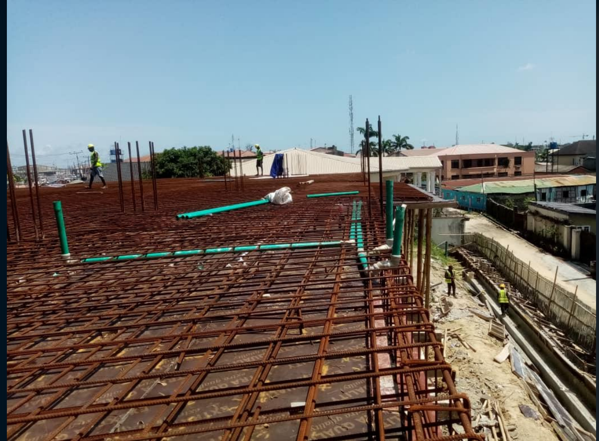
First Floor Slab Reinforcement Placement
