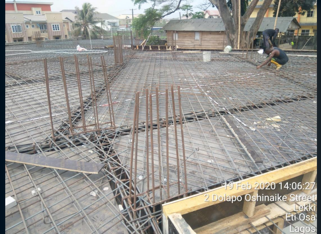
First Floor Slab Reinforcement Placement
