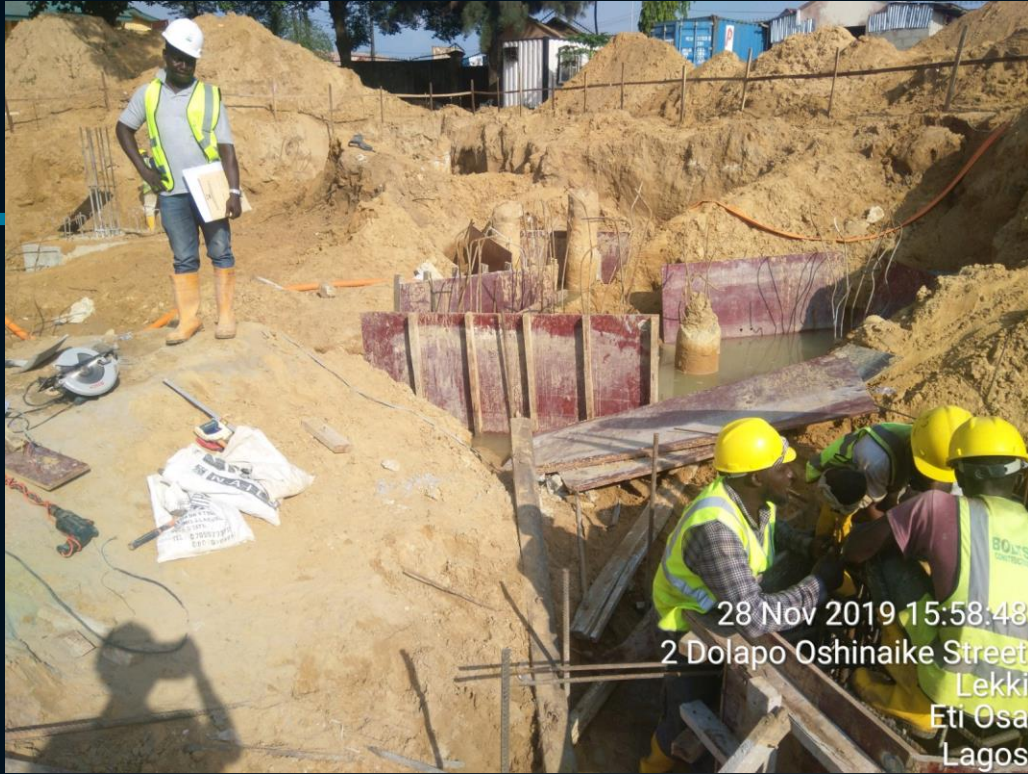
Construction of pile cap
