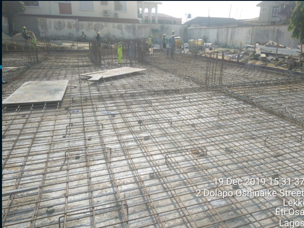
Raft slab reinforcement placement
