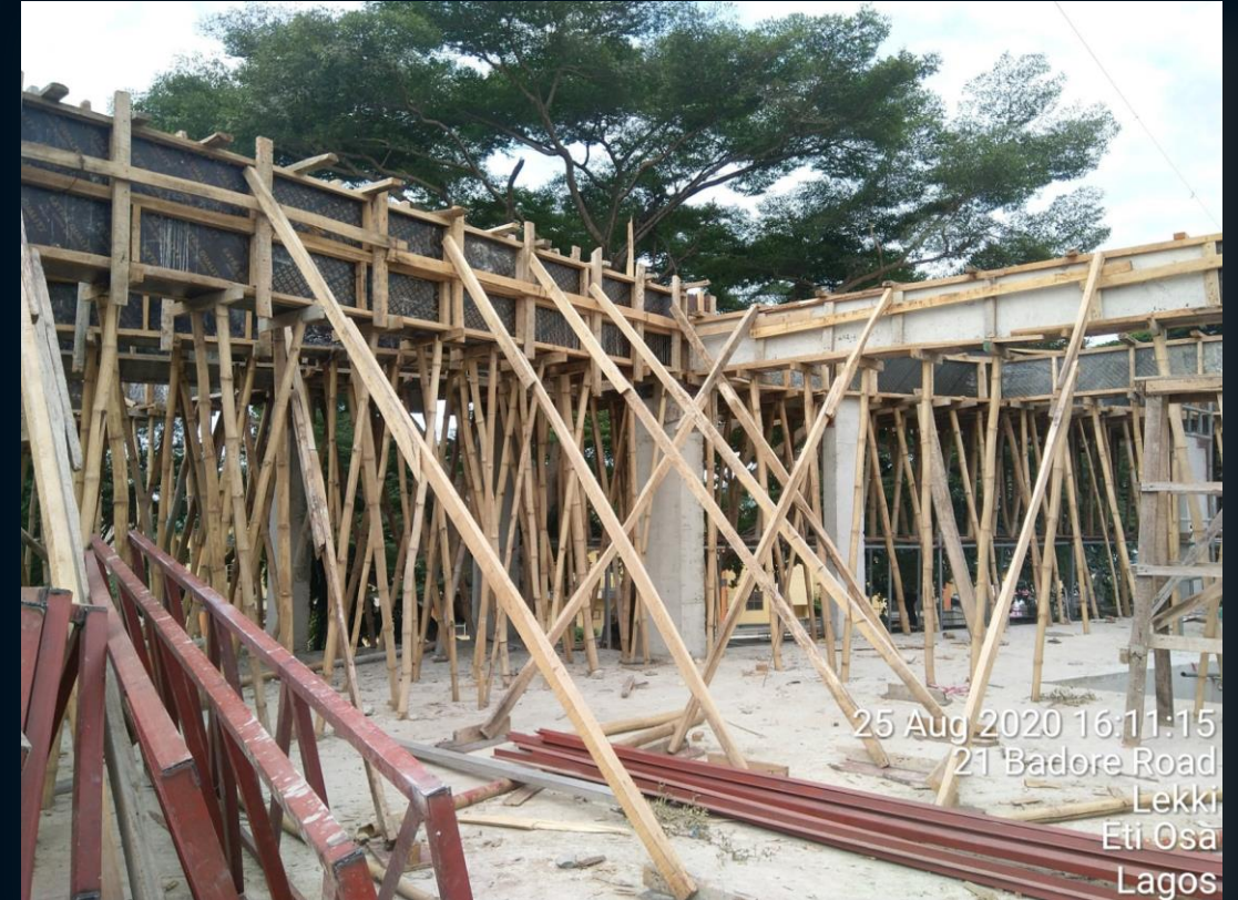
Roof Beams/Gutter Reinforcement placement
