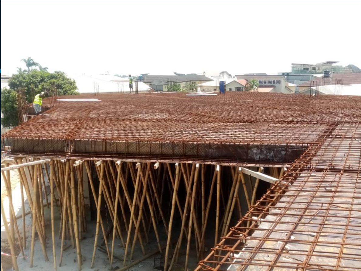
First Floor Slab Reinforcement Placement
