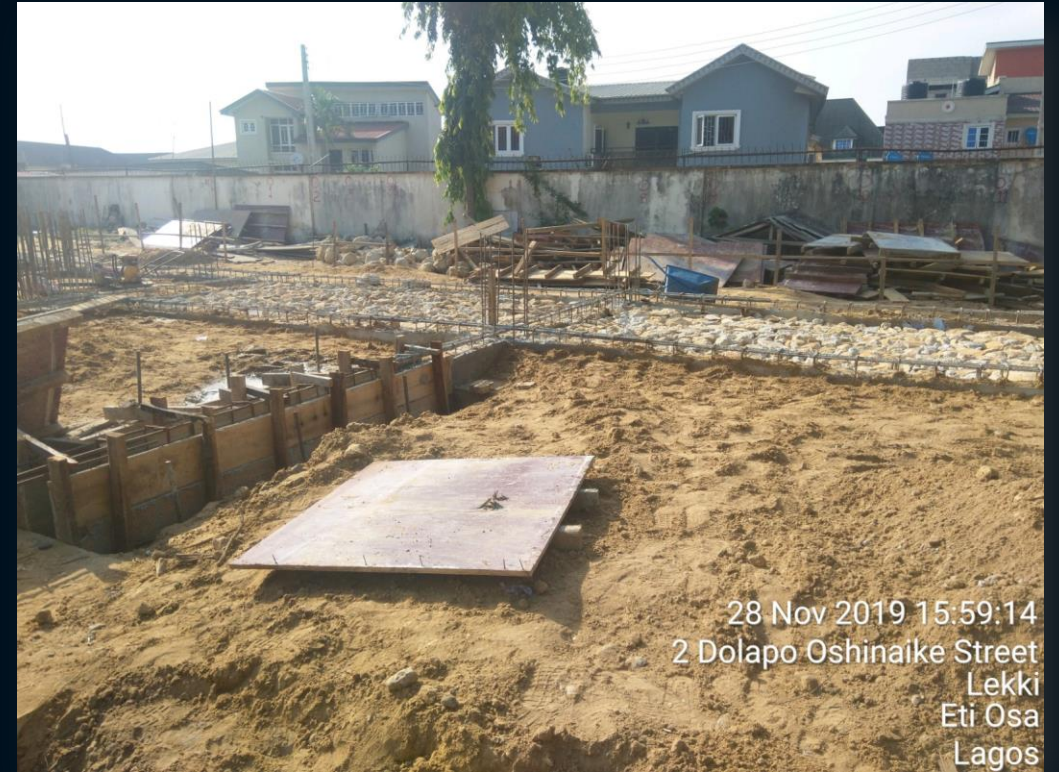
Construction of ground beams and backfilling
