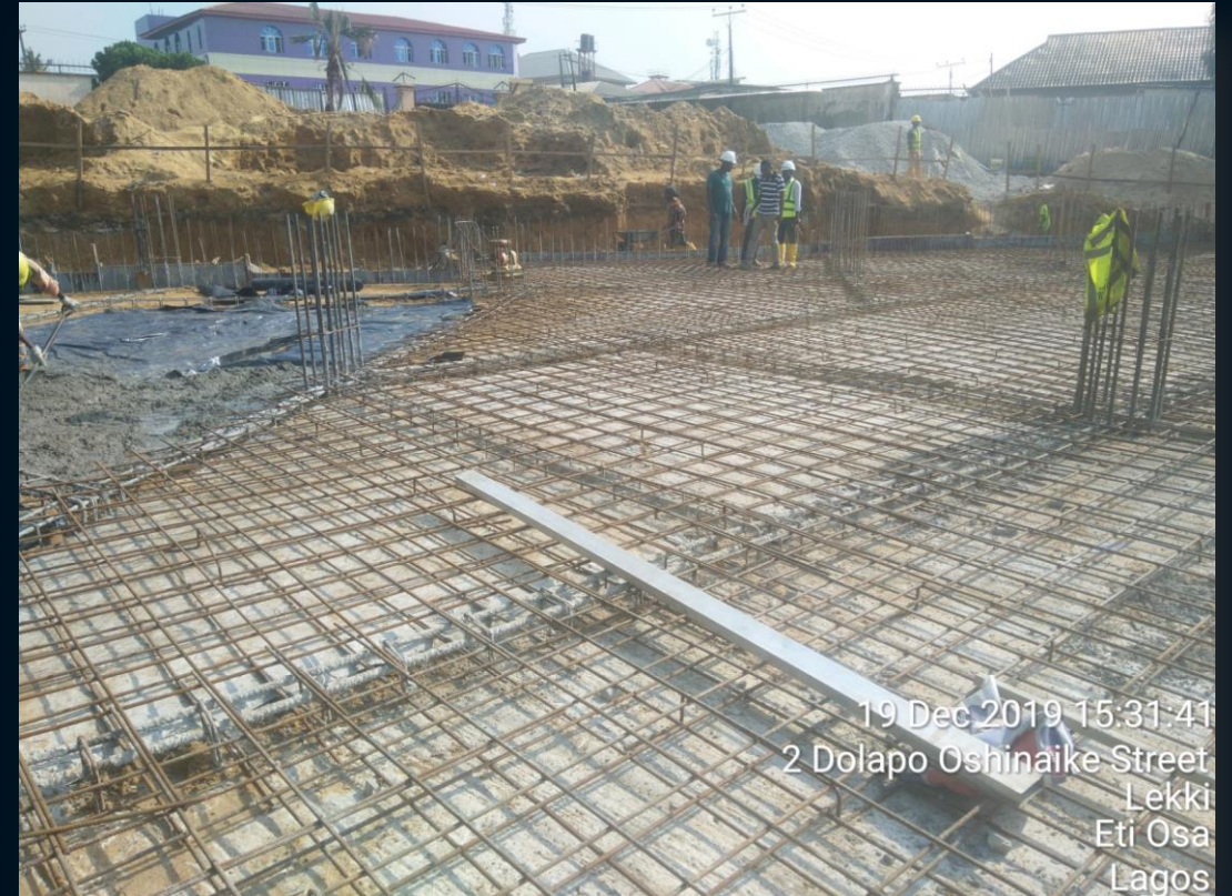
Raft slab reinforcement placement
