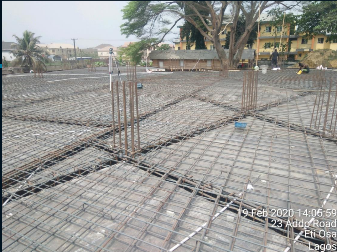
First Floor Slab Reinforcement Placement
