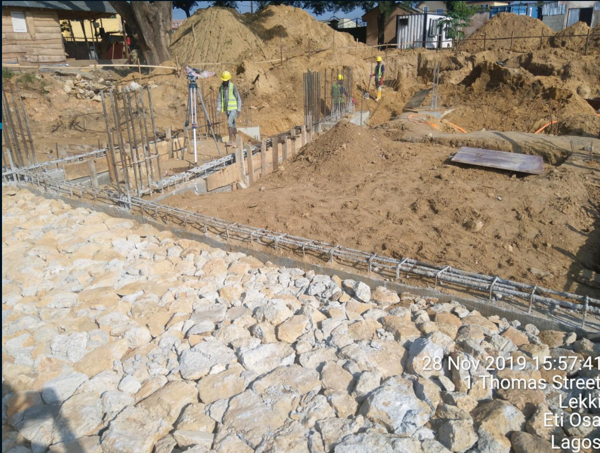
Construction of Ground beams and Backfilling
