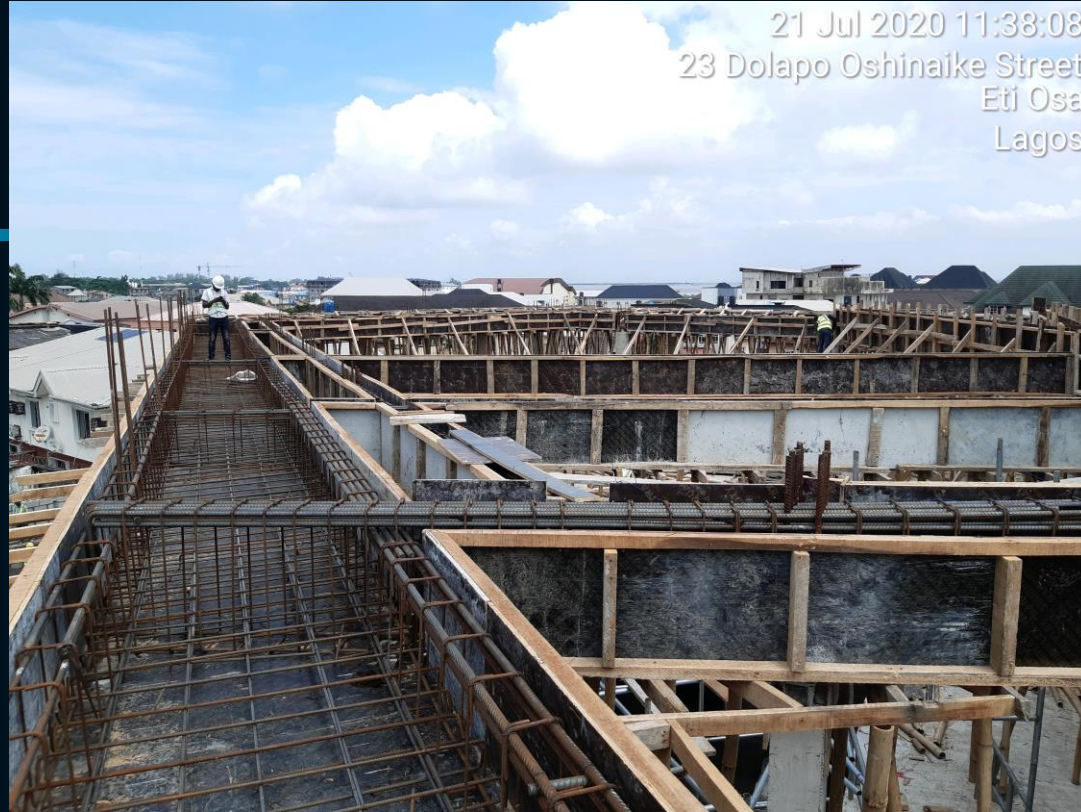
Roof Beams/Gutter Reinforcement placement
