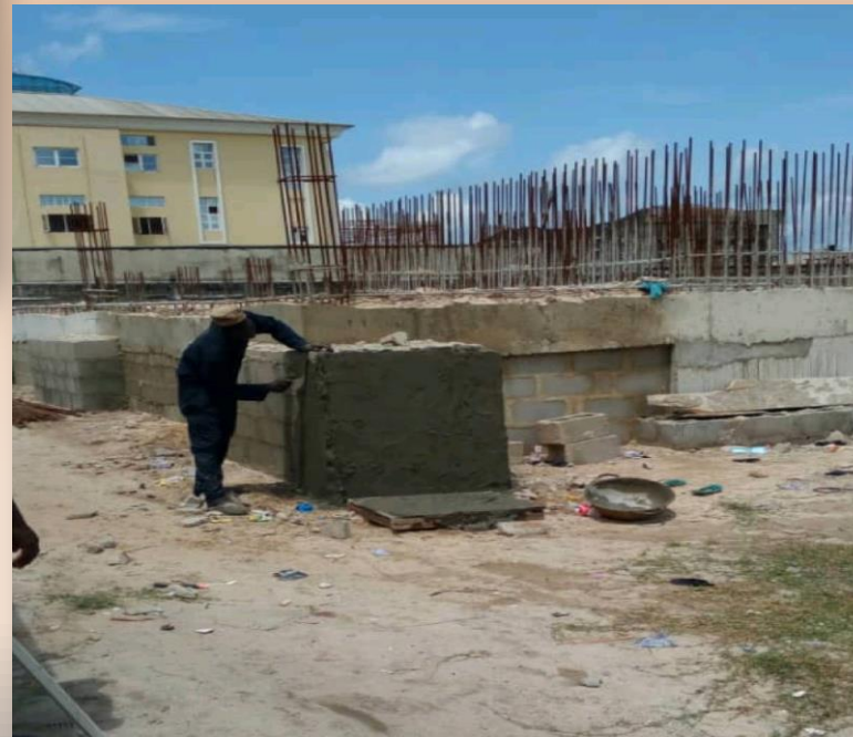
Concreting of ground beams
