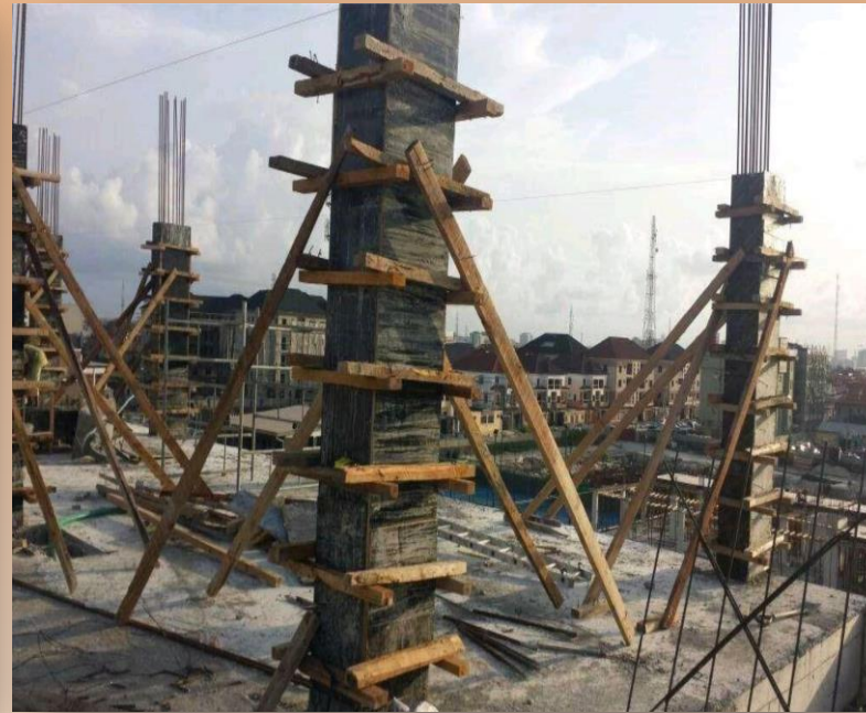
Construction of Upper floors Columns
