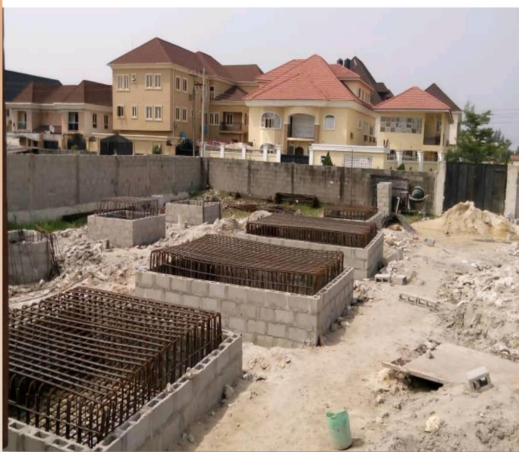
Reinforcement placement for pile caps
