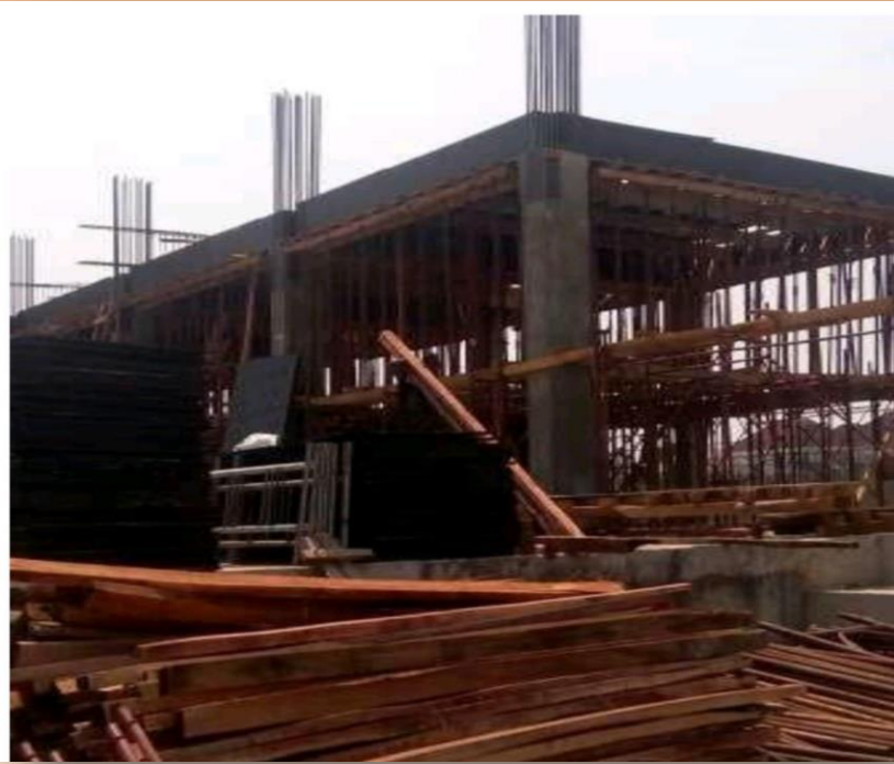
First floor formwork construction
