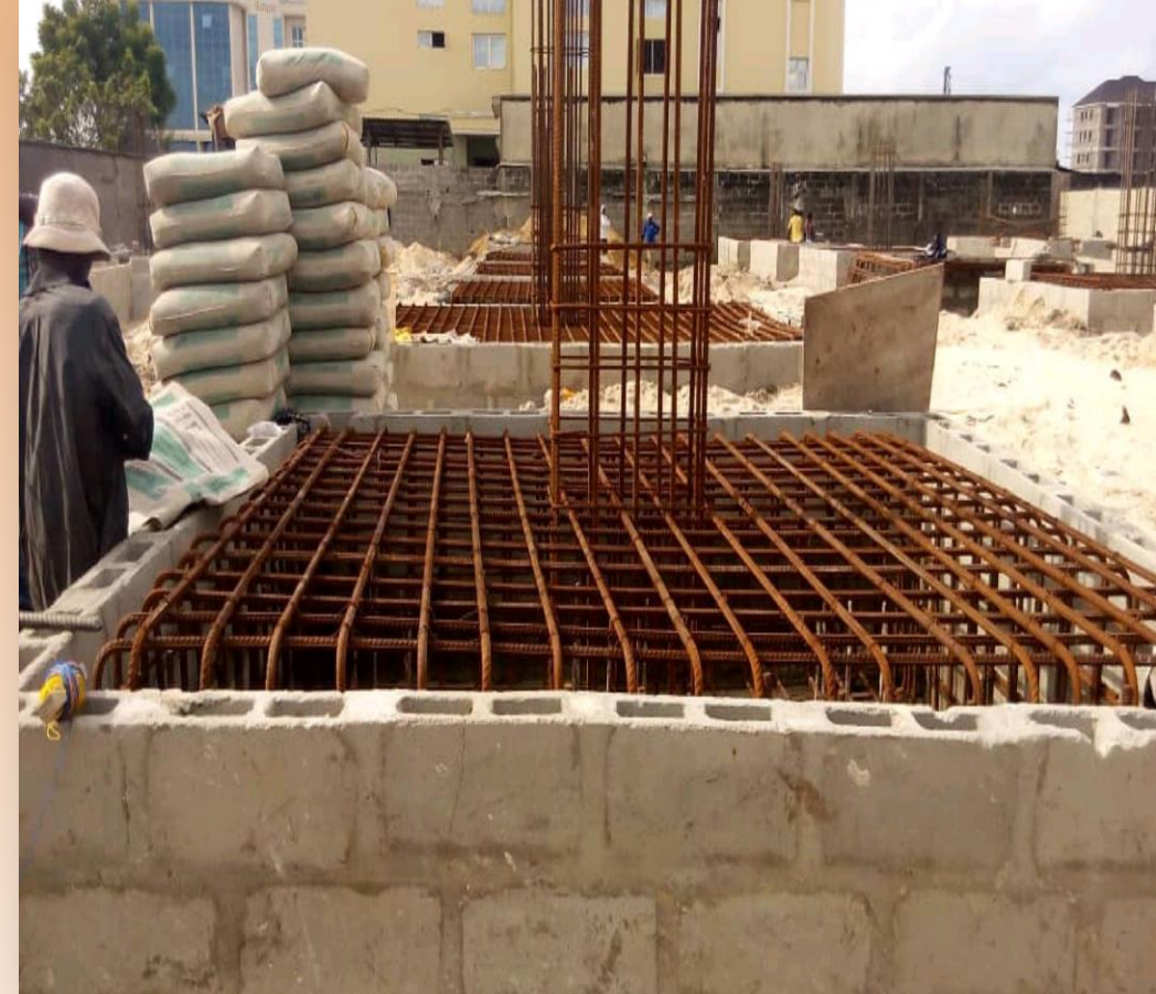
Reinforcement placement for pile caps
