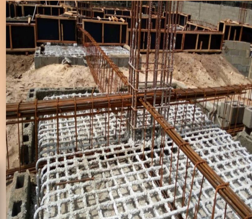
Ground Beams and Pile Caps Reinforcement placement
