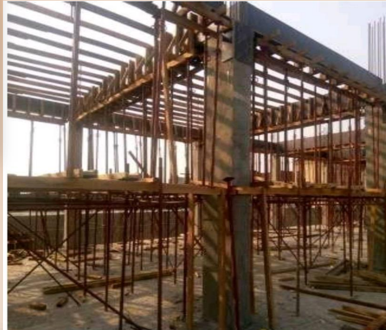
First floor formwork construction
