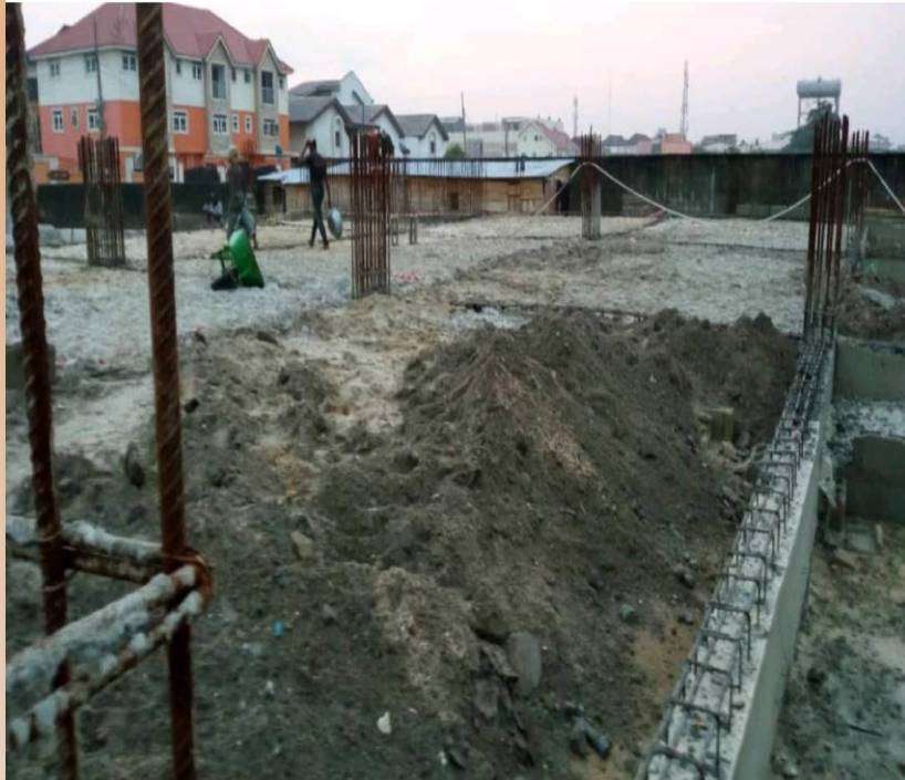
Ground Beams and Foundation Backfilling
