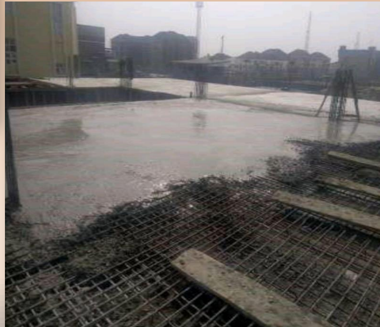
Concreting of Ground floor slab
