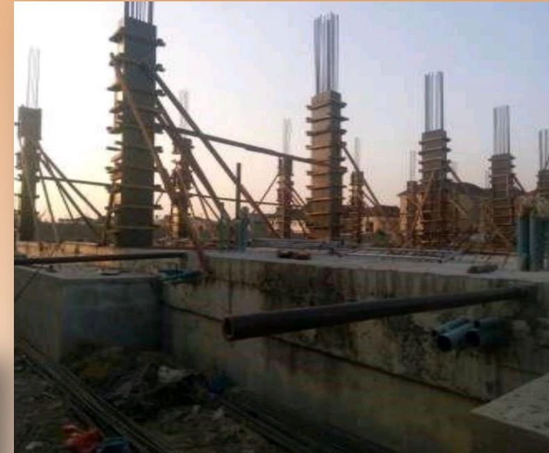
Ground floor columns formwork
