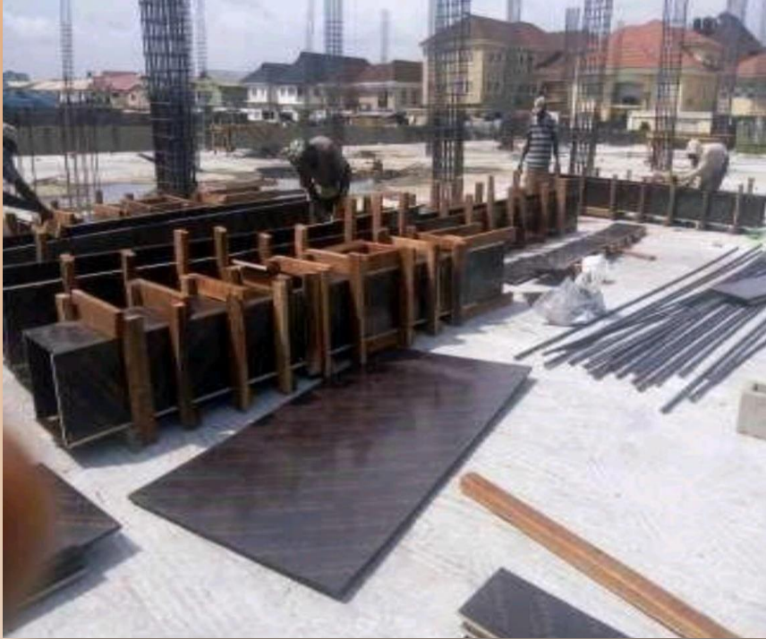
Placement of ground floor columns reinforcement
