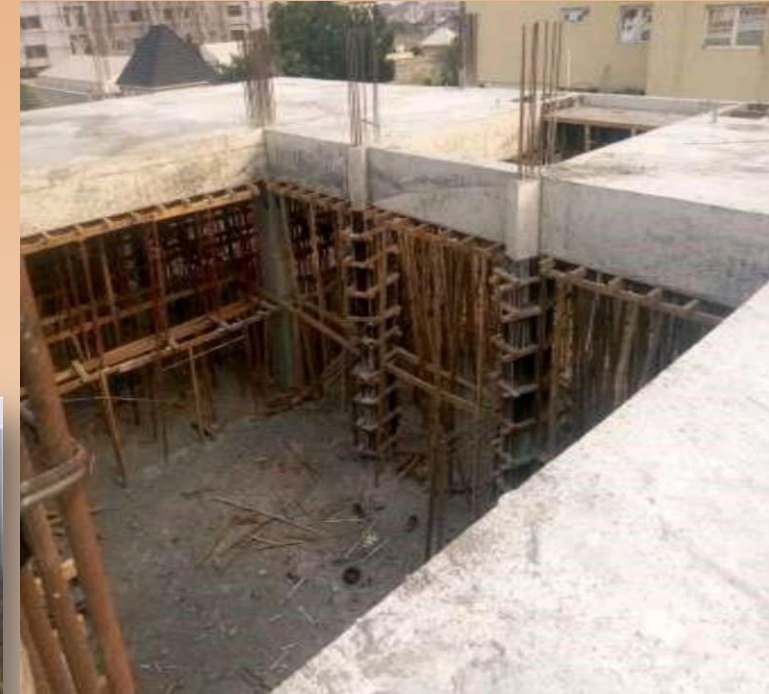
First floor concreting completed
