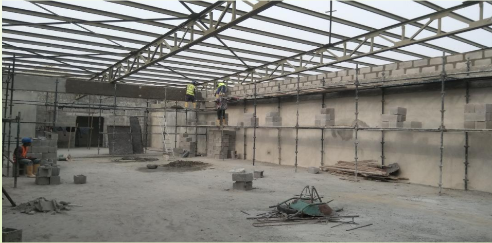
INSTALLATION OF ROOF TRUSSES
