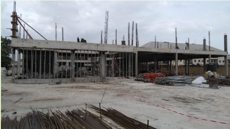
FIRST FLOOR SLAB AND BEAM REINFORCEMENT
