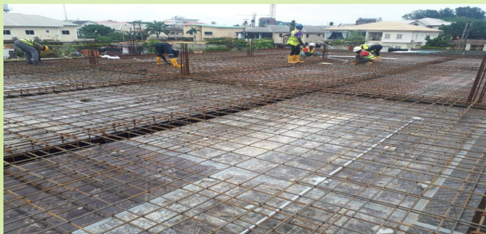
FIRST FLOOR SLAB AND BEAM REINFORCEMENT
