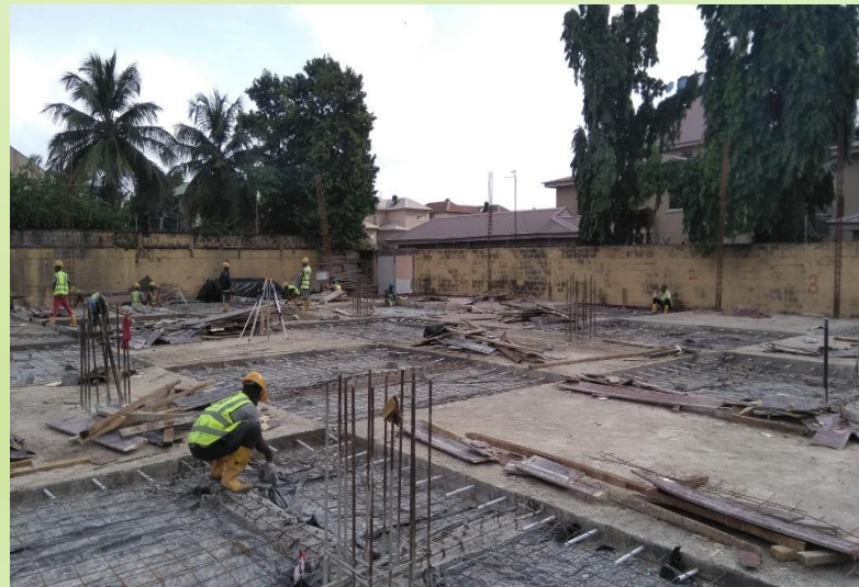
GERMAN FLOOR IRON REINFORCEMENT
