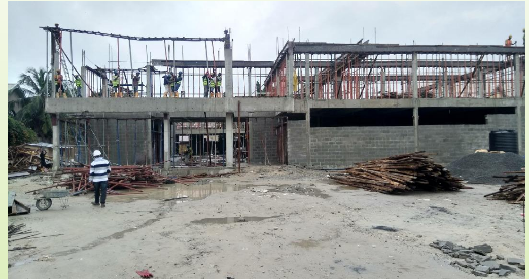
FIRST FLOOR COLUMN AND BEAM PREPARATION
