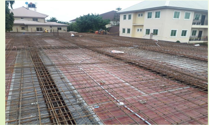
FIRST FLOOR REINFORCEMENT WORKS ONGOING
