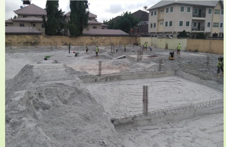
RAFT FOUNDATION CONCRETE WORK
