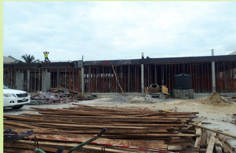
FIRST FLOOR DECK PREPARATION
