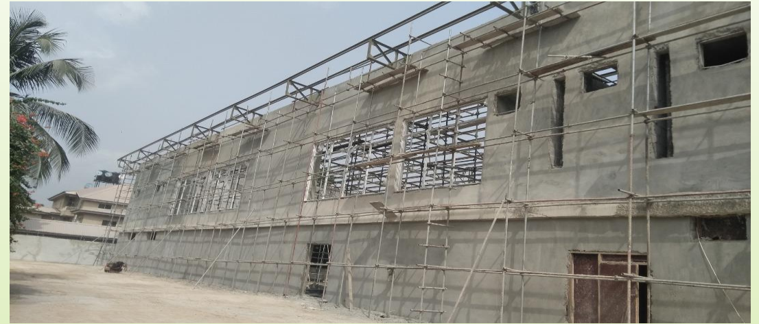
PLASTERING GOING ON
