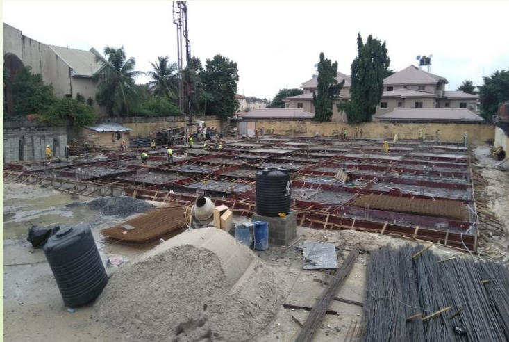
LAYING OF RAFT BEAM TO CONNECT CAP
