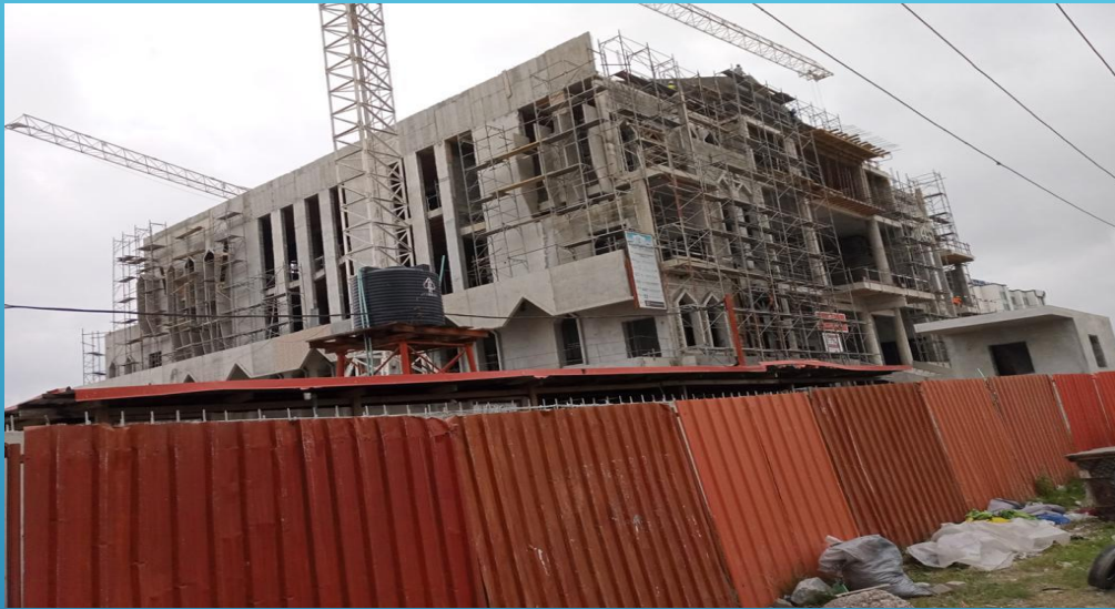
PLASTERING AND SCREEDING GOING ON.
