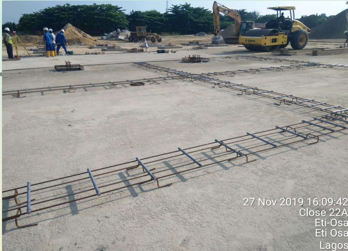
Installation of Dowel Bars for joints
