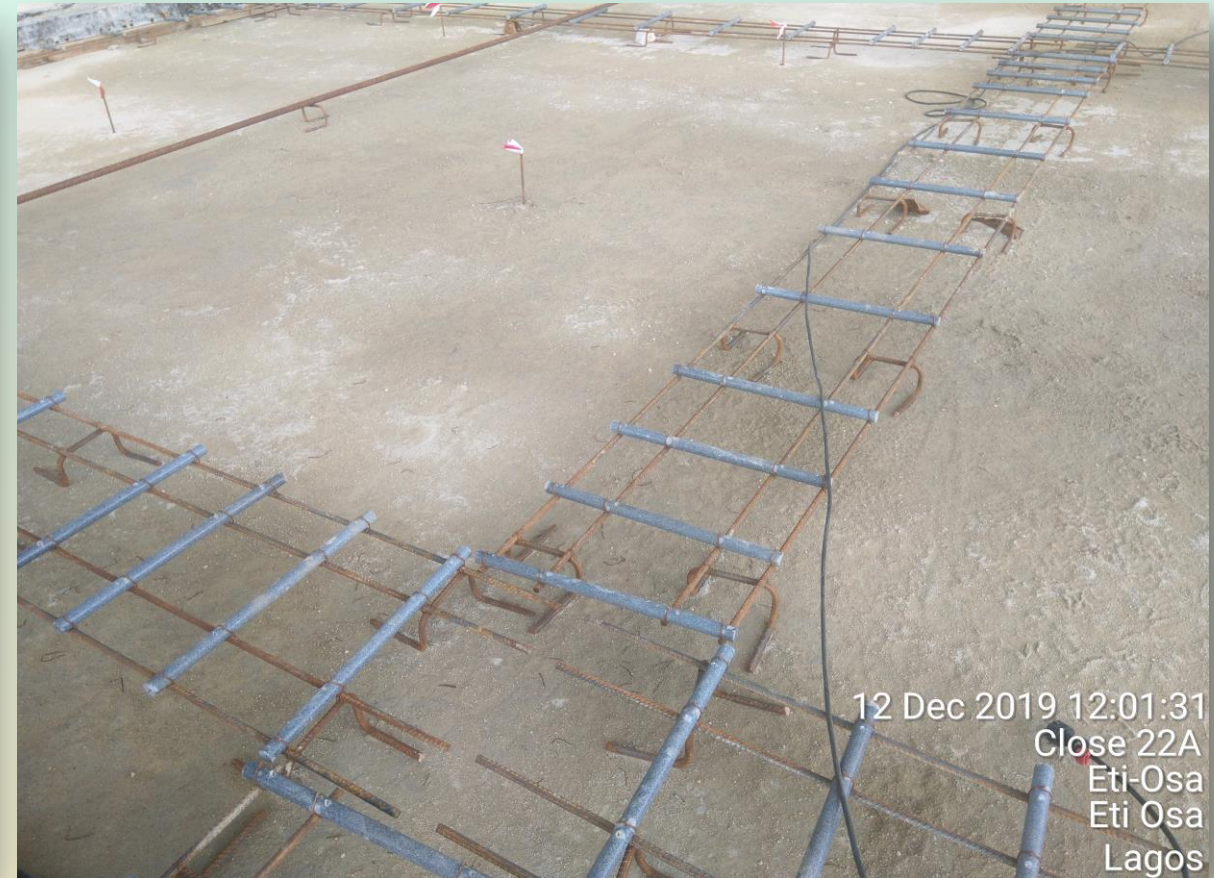
Installation of Dowel Bars for joints
