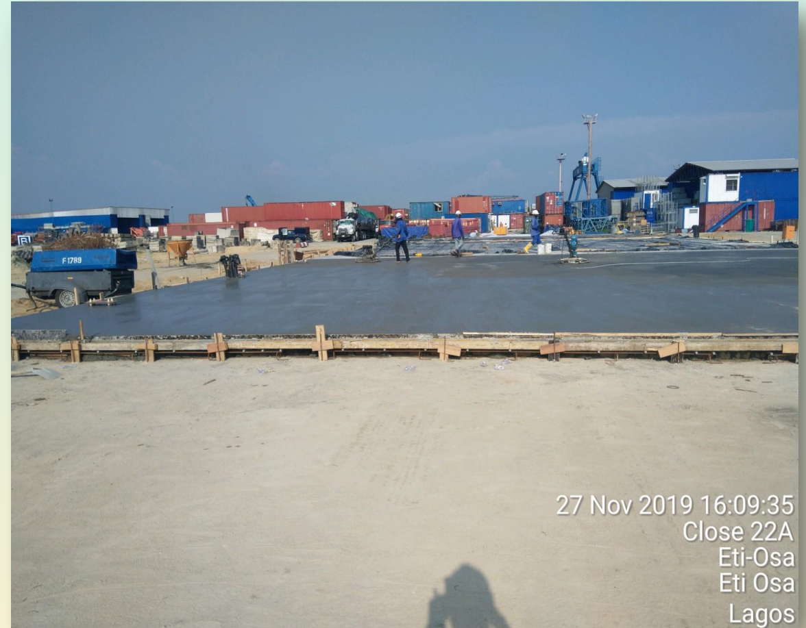
Concreting of Warehouse Pavement
