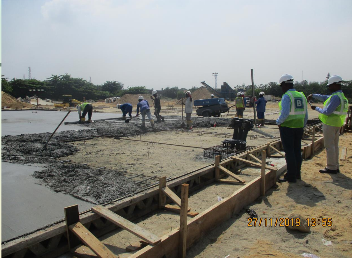
Concreting of Warehouse Pavement
