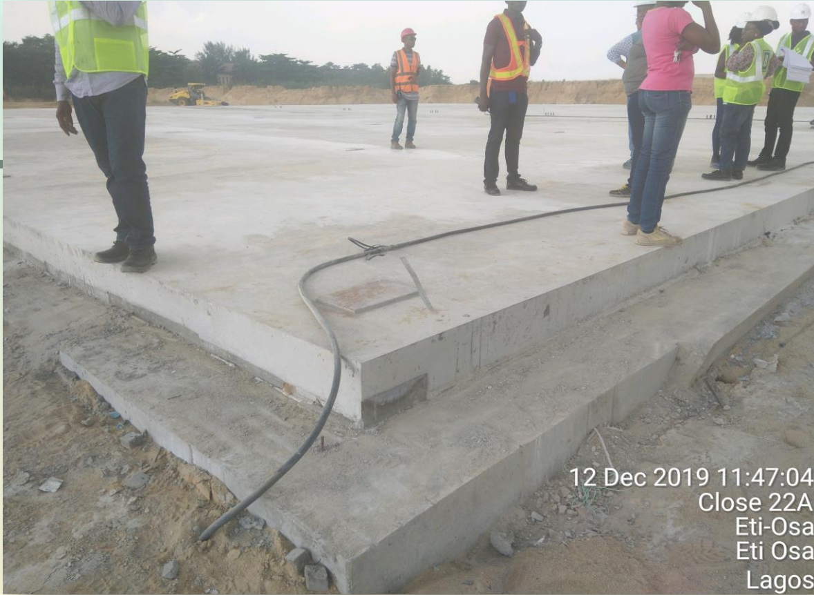
Completed Floor with Hold-Down-Bolt for Stanchion
