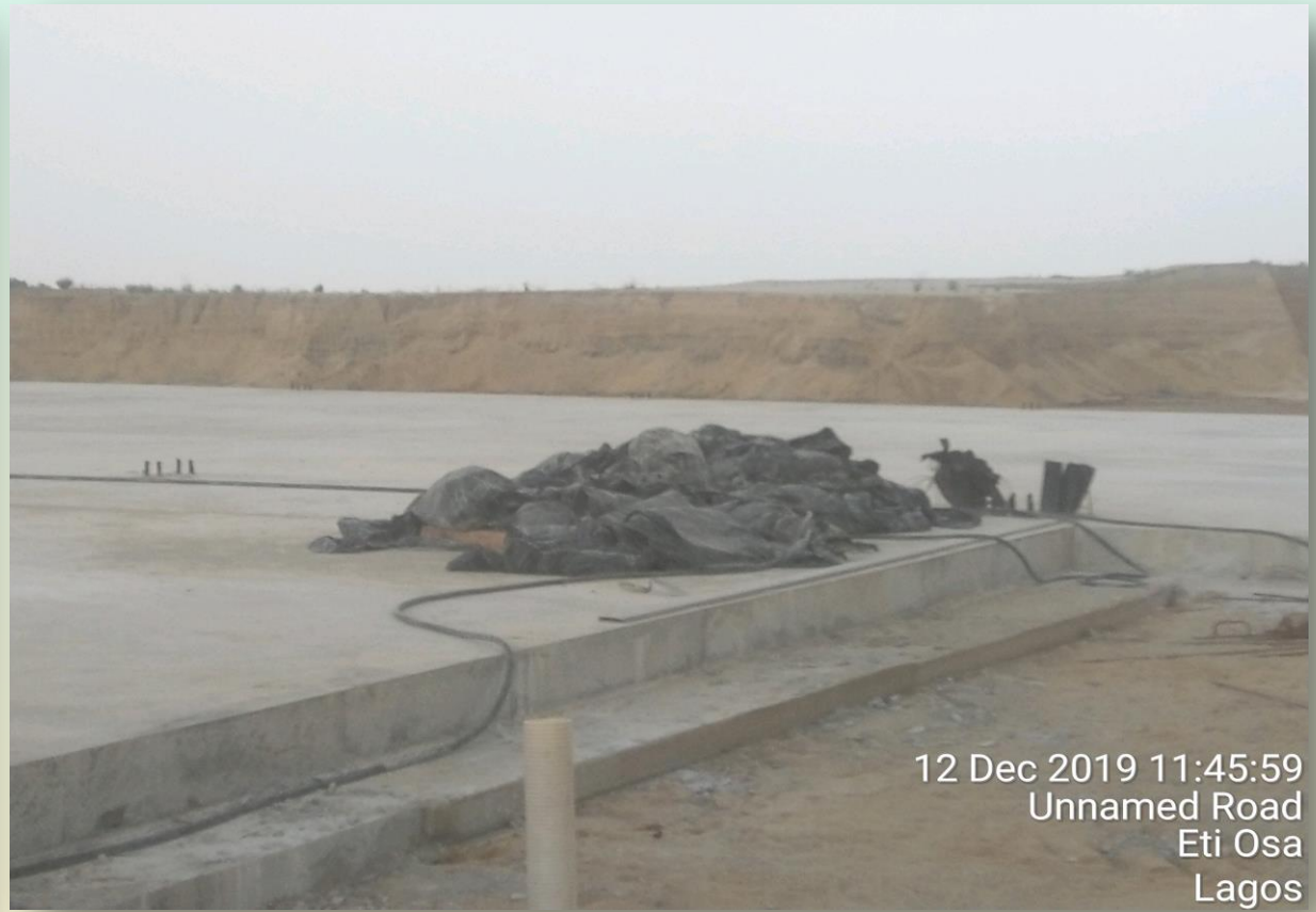
Completed Floor with Hold-Down-Bolt for Stanchion
