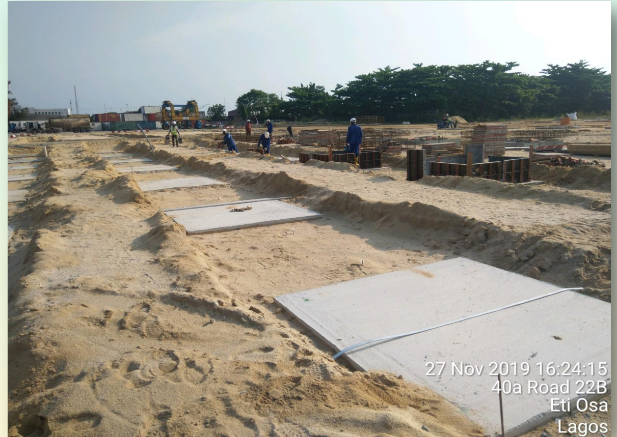
Foundation blinding for Stanchion Bases
