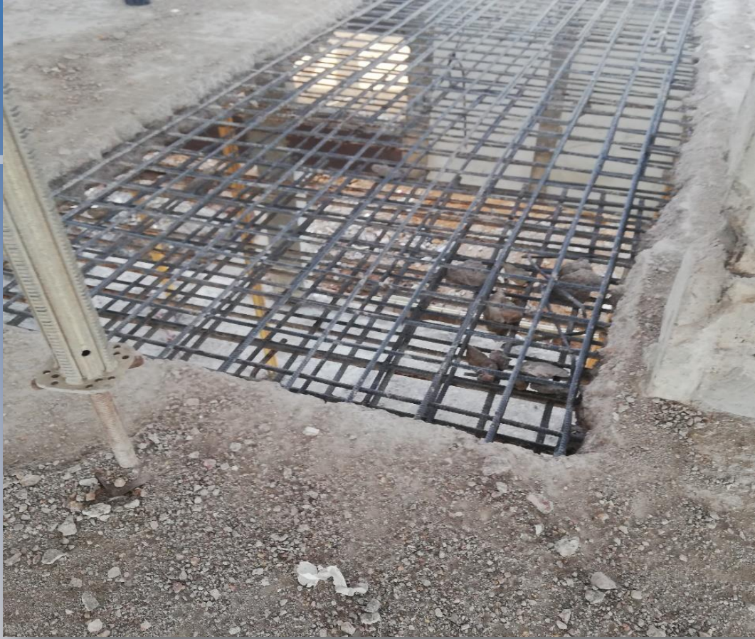
Placement of reinforcement for foundation of new structure
