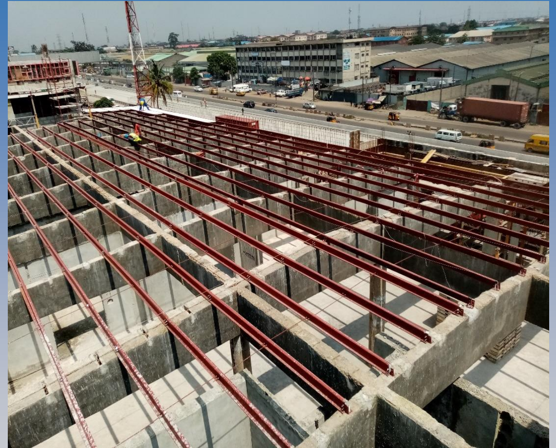
Installation of roof trusses
