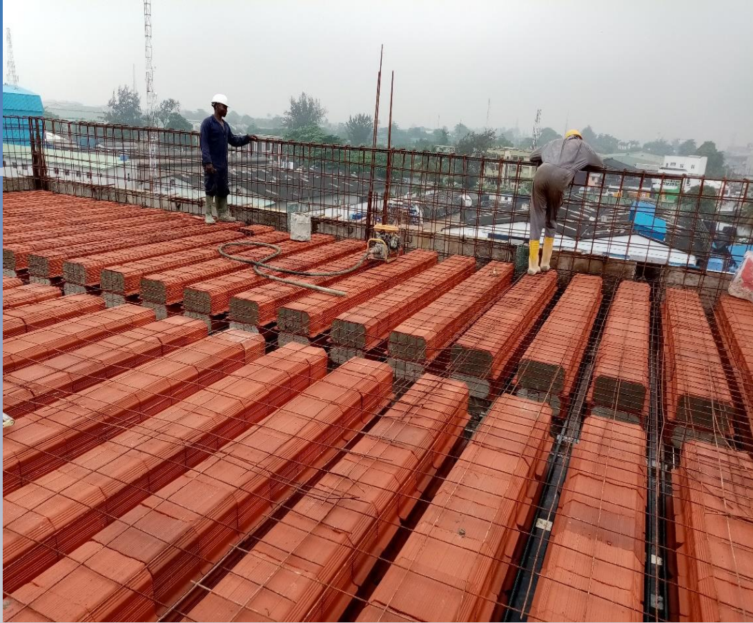
Construction of new suspended floor
