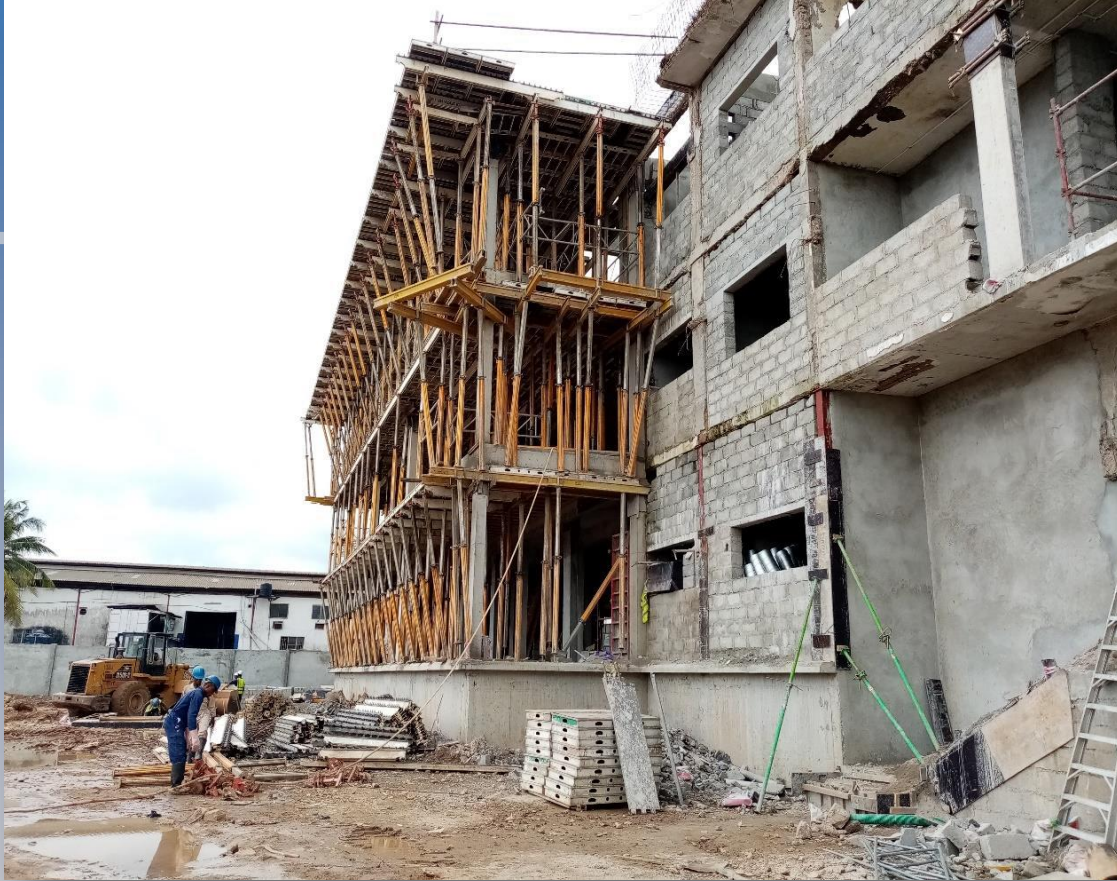
New blockwork and structural framework
