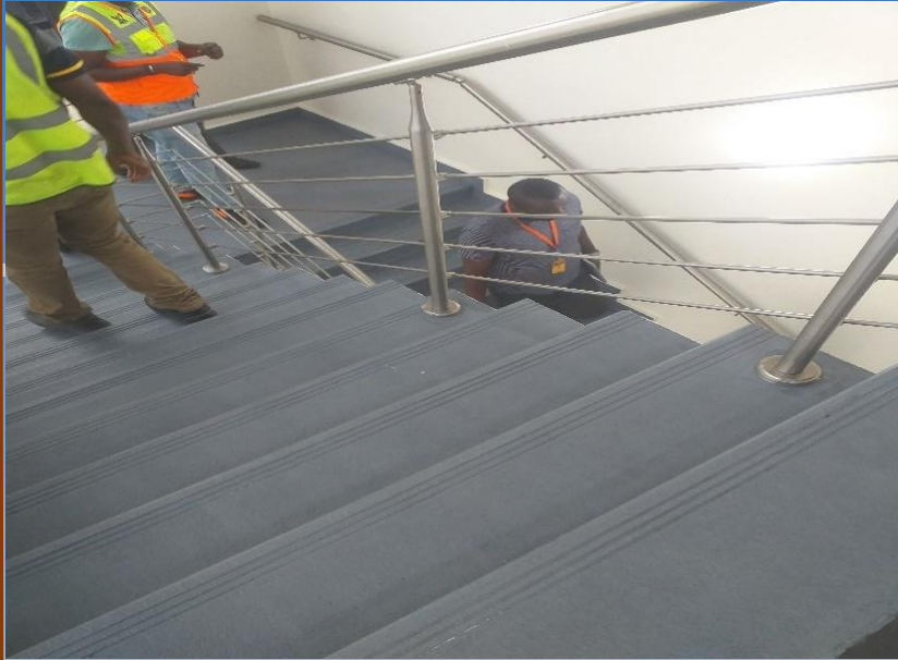
Internal finishes of the structure
