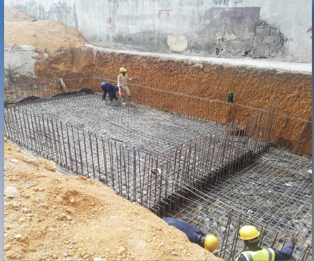
Placement of reinforcement for foundation of new structure
